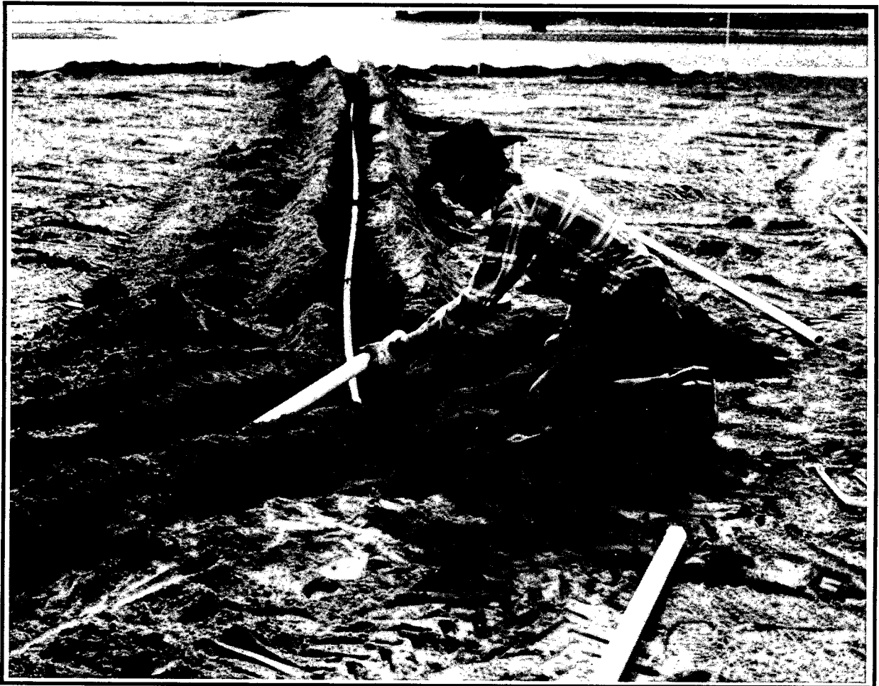
Sometimes turf areas are so compacted and the irrigation system so corroded that it is best to tear out the old and start fresh.
