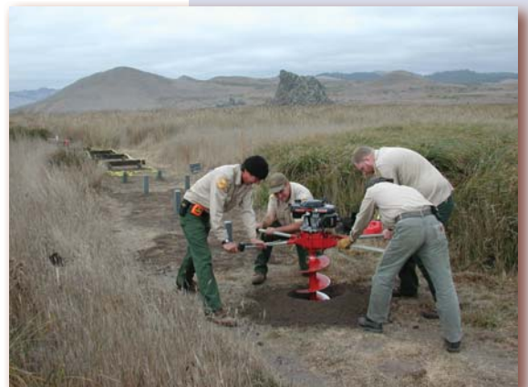
Trail construction at California State Parks
