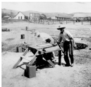
Molding adobe tiles and bricks for the redevelopment of the Casa de Estudillo into Ramona’s Marriage Place.
