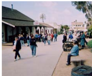
A concrete road rings the plaza, detracting from the historic environment.
