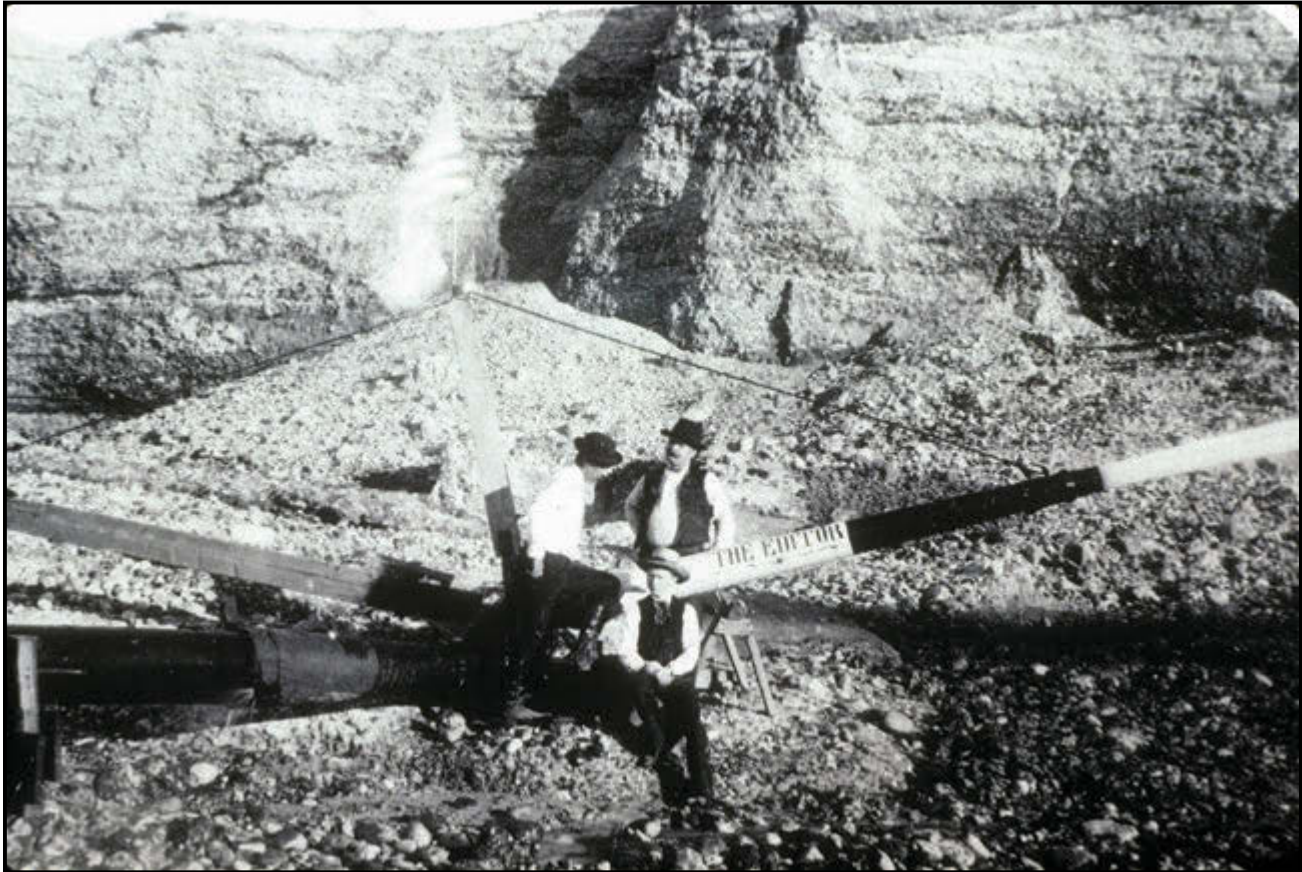
Figure 7. Miners pose in the Pit in front of a water monitor dubbed “The Editor”, ca. 1880s. Historic Slides, MDSHP Collection.
