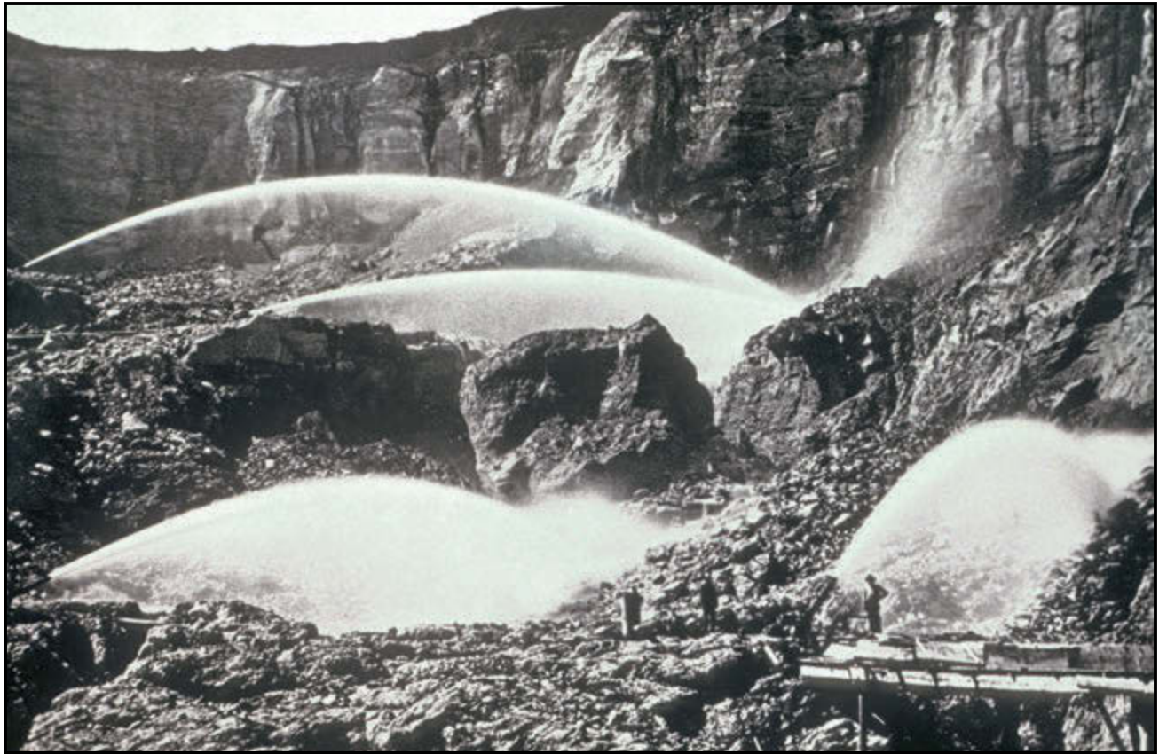
Figure 5. Giant water monitors working in the Pit, Historic Slides, MDSHP Collection.
