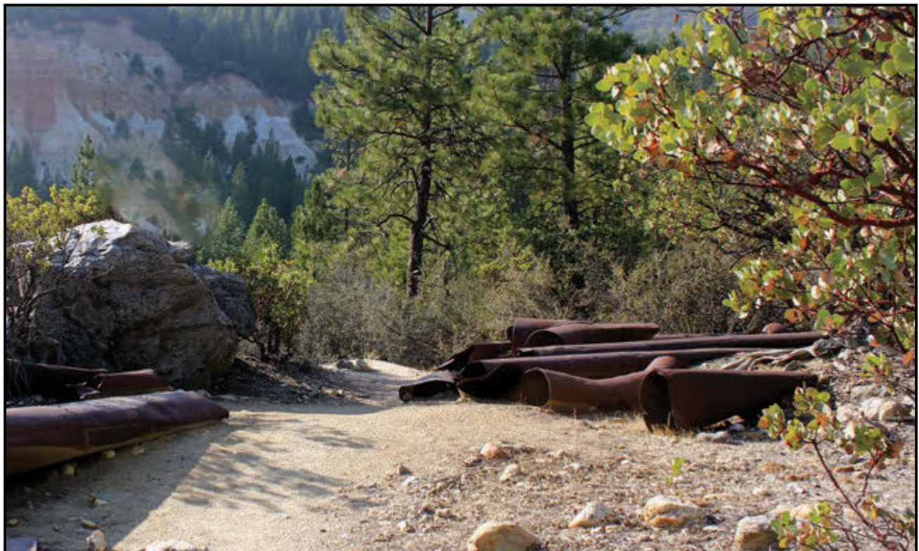
Figure 24. The Diggins Loop Trail cuts through remnants of the hydraulic mine's water conveyance system, 2013.
