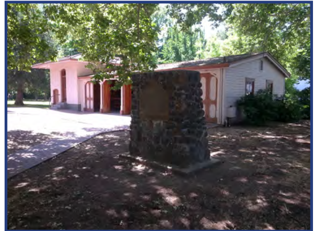
Architect's Cottage, Carriage Shed, and Historical Marker.
