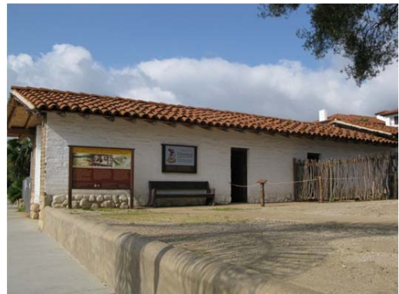
Portion of Northwest Corner
