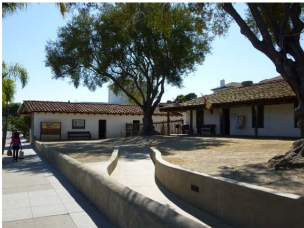
A new accessible entrance and restroom were constructed as part of the Northwest Corner project (the Canedo Adobe is on the right).
