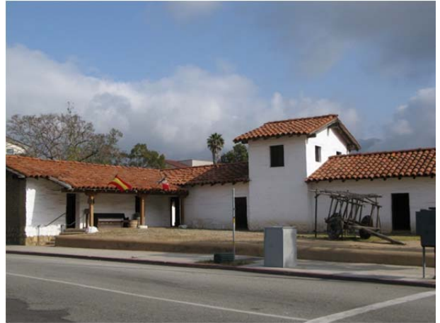
The buildings of the Santa Barbara Presidio, including the reconstructed Northeast Corner shown here, display the white-washed adobe walls and red tile roofs typical of Spanish colonial settlements in Alta California.
