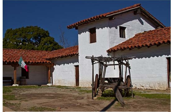
Northeast Corner Complex
