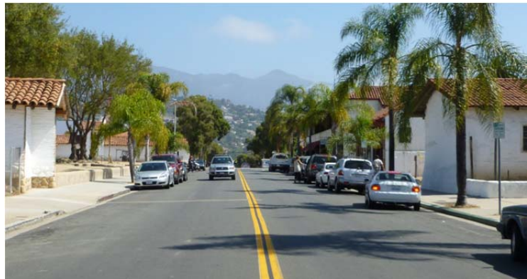
Visitors entering El Presidio SHP on Canon Perdido Street pass El Cuartel (right) and the newly reconstructed Northwest Corner (left). Limited street parking is available. A public parking structure is a block away.
