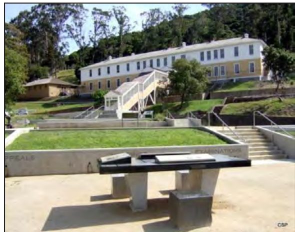
Figure 19. Restored USIS Detention Barracks with new accessible paths
