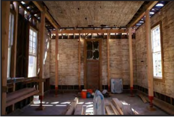
Figure 9. USIS Hospital Ward rehabilitation, c. 2011
