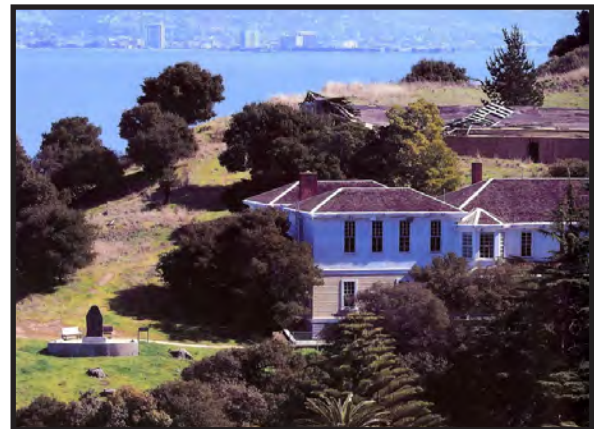
Figure 8. USIS Hospital, c. 2011
