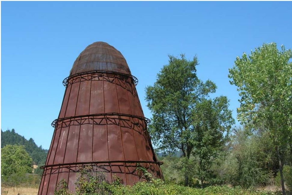
Figure 103. Abandoned "tipi burner." Such burners, once used to dispose of sawmill waste, were common until the 1970s. Now the wood that was formerly wasted has many uses, and the air pollution from burning waste is not allowed. See also Figure 102. (Photo by Michael Roa.)
