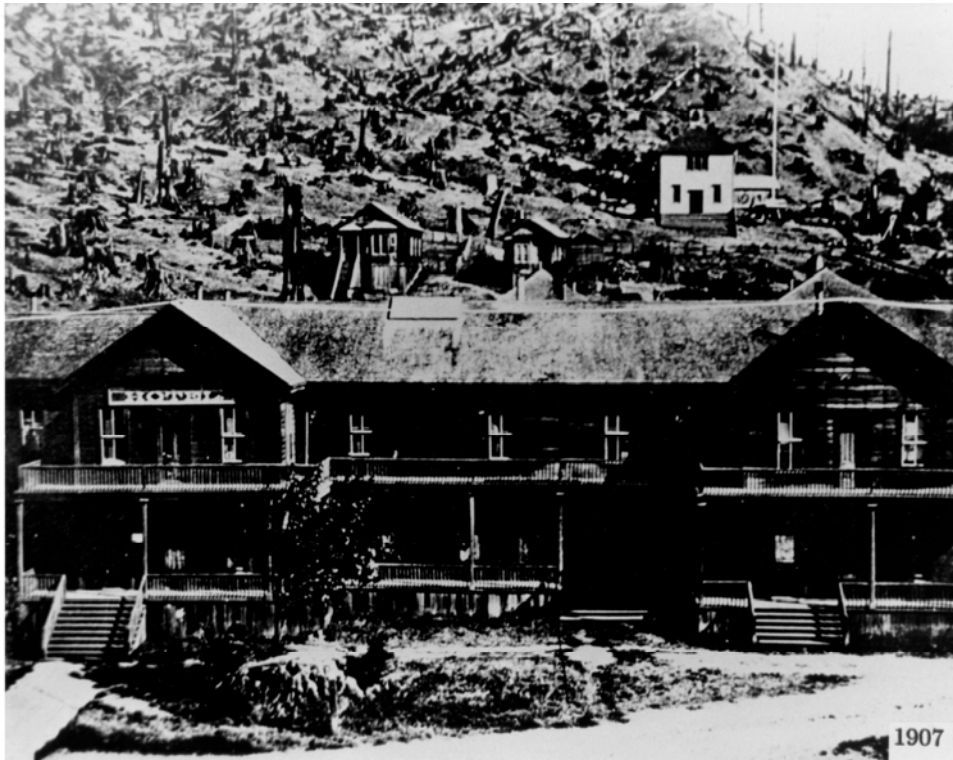
Figure 105. The Scotia Inn (Hotel) in 1907. Compare the hillside in the background to the regrown hillside circa 1970s-1980s (Figure 106). (Photo courtesy Pacific Lumber Company.)
