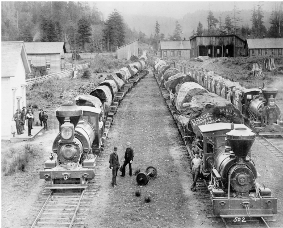
Figure 90. Railroad trains were often used to move logs to the mills. Scene at Freshwater in 1890. (Photo courtesy Pacific Lumber Company.)
