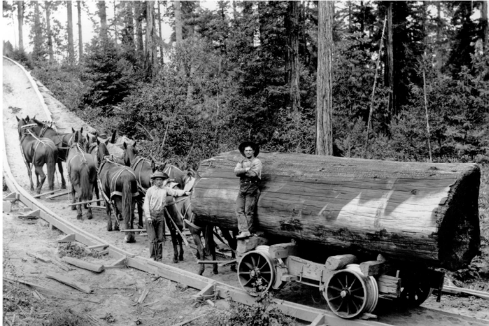
Figure 89. Temporary horse- or mule-drawn "railroad" with wooden tracks. Sometimes logs were used for tracks instead of boards. Note the wide wheels on the cart. (Photo courtesy of the California Redwood Association.)
