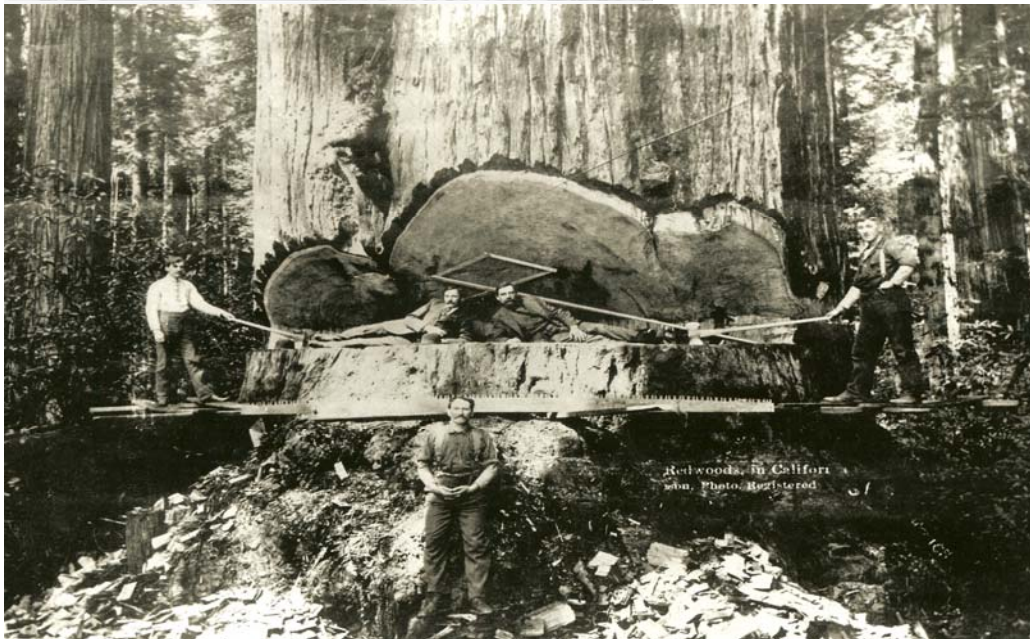
Figure 79. Logging with axes was hard, dangerous, time-consuming work. To fell the large trees, special axes with longer handles were made. The introduction of the whipsaw made the felling of the giants easier and faster. (Photo courtesy Clarke Museum.)
