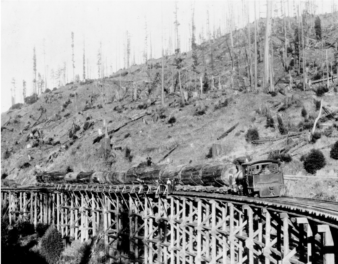
Figure 88. The rugged terrain of northern California required the building of some impressive railroad trestles. Note the nearly clear-cut hillside, and also that young trees have started to grow. For scale, see the man standing on a log near the middle of the train. (Photo courtesy of Pacific Lumber Company collection.)
