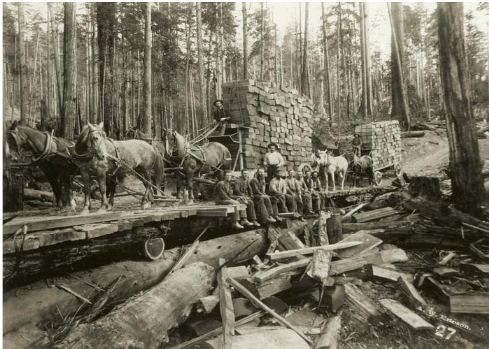
Figure 87. Shingles and boards were needed for building houses. Redwood's resistance to rot made it ideal for shingles, grape stakes and railroad ties. Here "split product," probably shingle wood, is moved by horse-drawn cart to a shingle mill, port or railroad loading area. (Photo courtesy Clarke Museum.)
