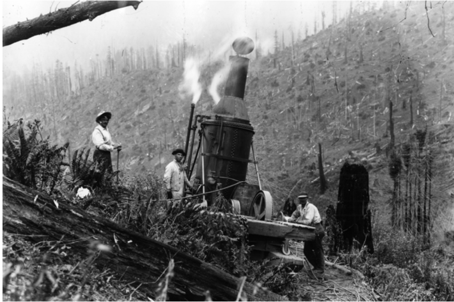
Figure 84. The Dolbeer Donkey engine, named for its inventor, John Dolbeer, a partner in the Dolbeer and Carson Lumber company of Eureka, made it easier and faster to move logs to a landing. It also was harder on the forest plants and forest floor. (Photo courtesy Humboldt State Library Humboldt Room collection.)
