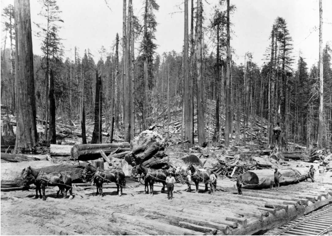
Figure 82. Teams of mules or horses were used to drag logs to the rail landing, or to a river. Skid trails of logs were made to keep the logs from digging into the ground. Many trees were often left standing because only the best trees were cut. (Photo courtesy of Pacific Lumber Company collection.)
