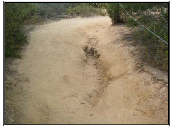
Erosion gully on Beach Trail
