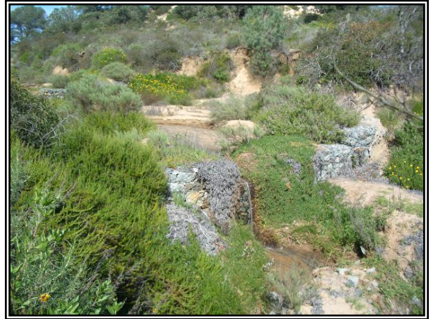
Drainage channel at Mar Scenic Trail with weir
