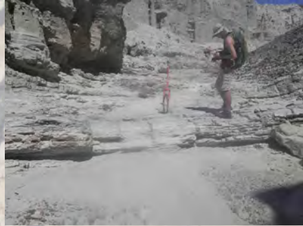
Photo 6924. Improper Grade. Barrier to vehicle passage. High
