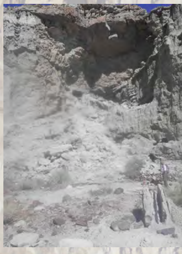
Photo: 6919 Unstable Slope, sliding banks. Critical
