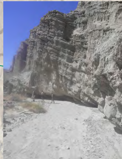
Photo: 6926. Unstable slope. High
