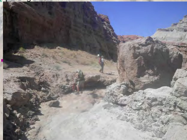
Photo: 6934. Improper grade. Barrier to vehicle passage. Critical
