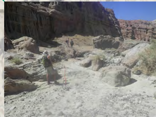
Photo 6932. Unstable slope, sliding banks. High
