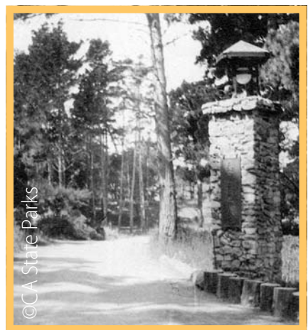
Asilomar entry pillar, 1925
