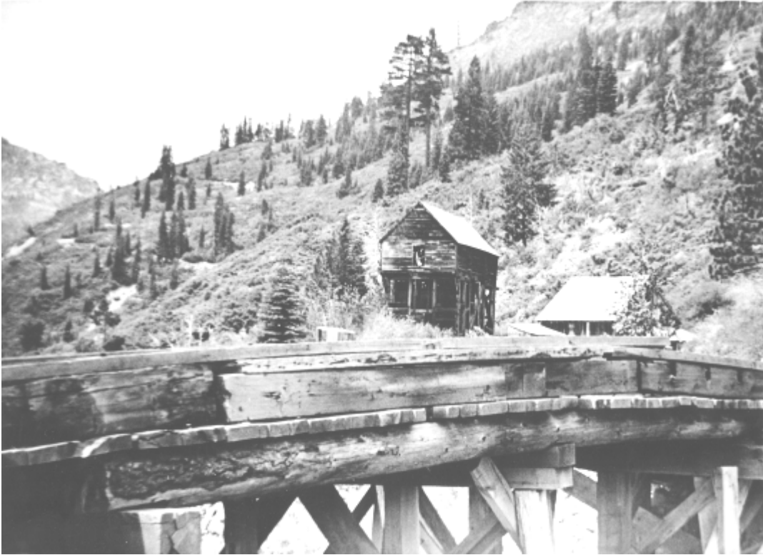
Ore cart trestle to the Mohawk Mill with the tram terminus building in background, aerial tram from the 76 mine... closed for the season
