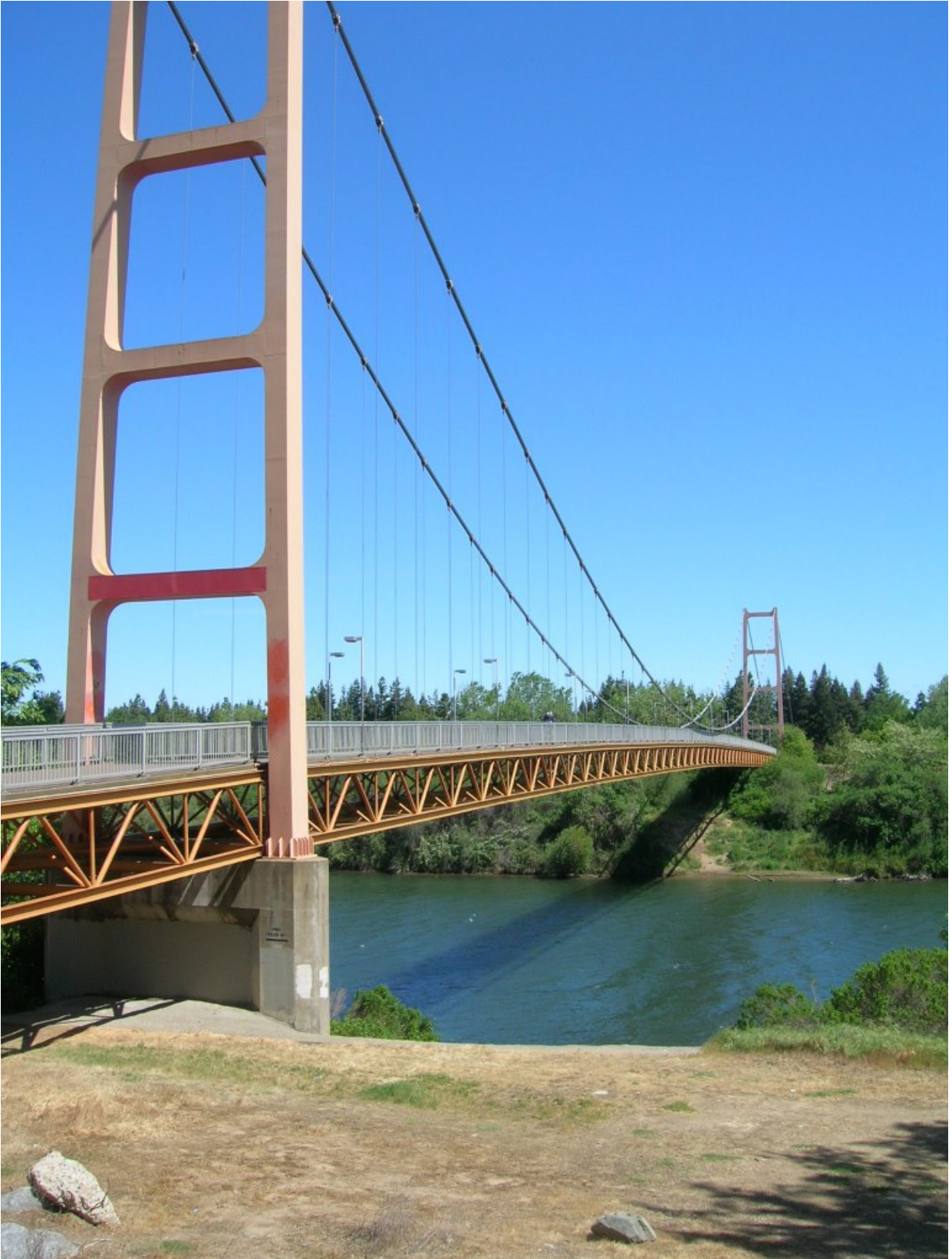
Figure 9 Suspension Bridge with Towers and Support Truss Below Deck
