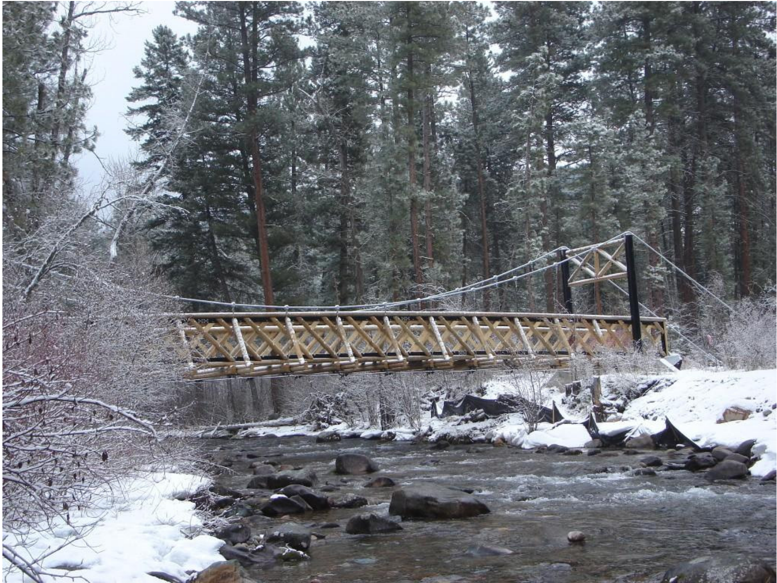
Figure 10 Suspension Bridge with Towers and Support Truss above Deck
