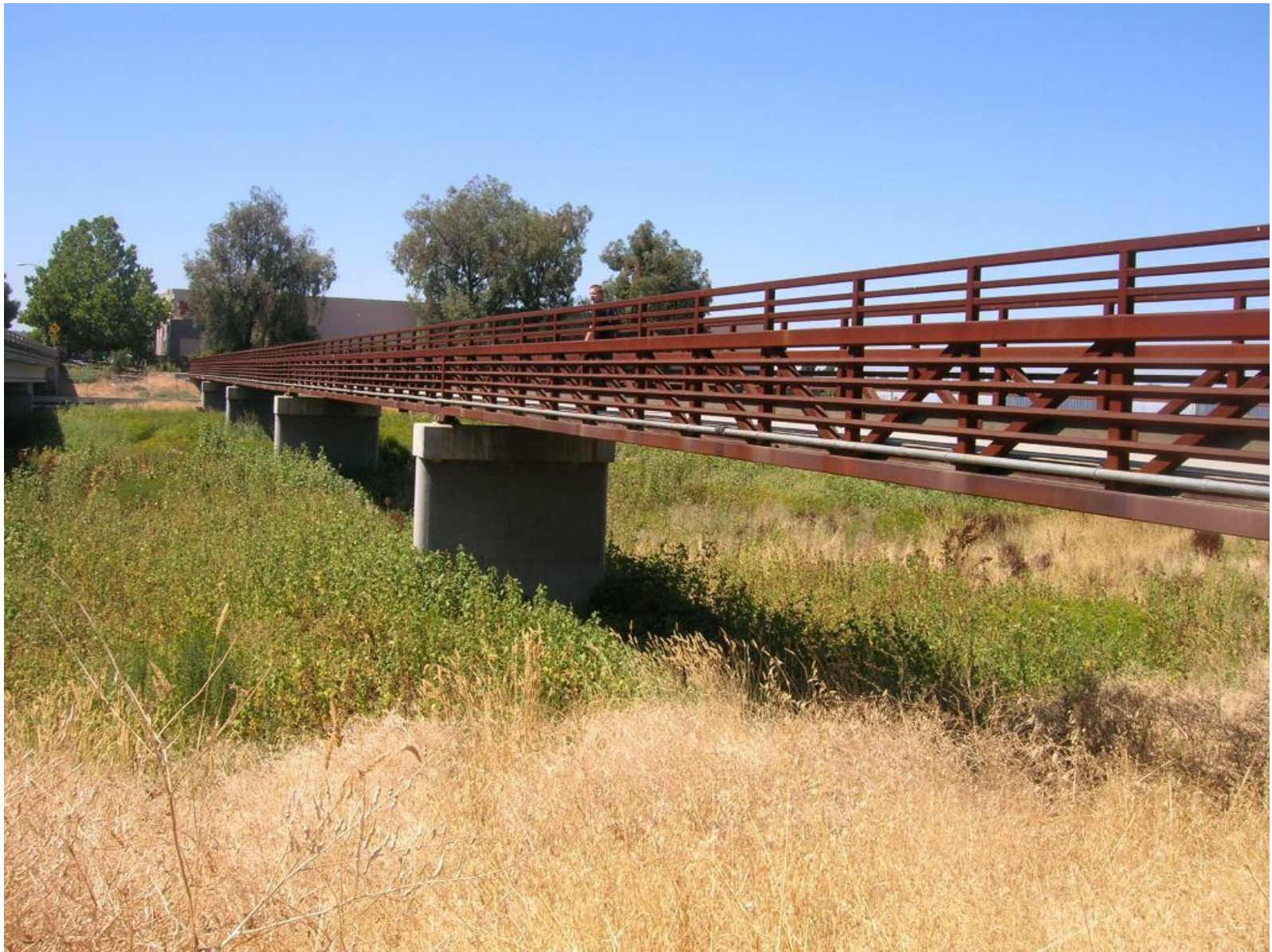
Figure 7 Prefabricated Steel Truss
