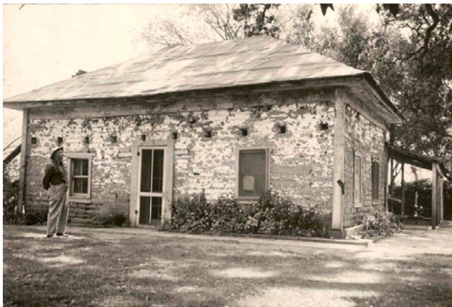
George Sutton stands next to the house he helped make a state park. Note the attachments embedded in the adobe walls for the veranda roof—now missing. California State Parks Collections.
