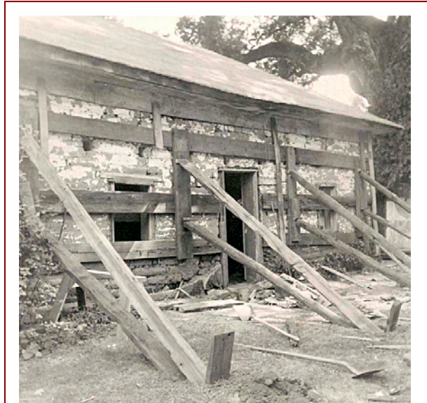
Exterior shored walls of the Adobe in July 1958. California State Parks Collections.
