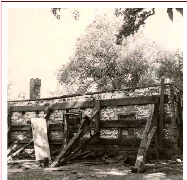
The Adobe after the roof was removed in July 1958. California State Parks Collections.
