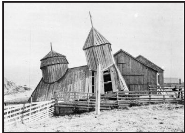
Figure 3. The RAC-era chapel collapsed during the 1906 earthquake, CSP 090-4727 .
