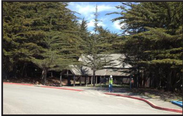
Figure 30. Overgrown cypress trees obscure the building.
