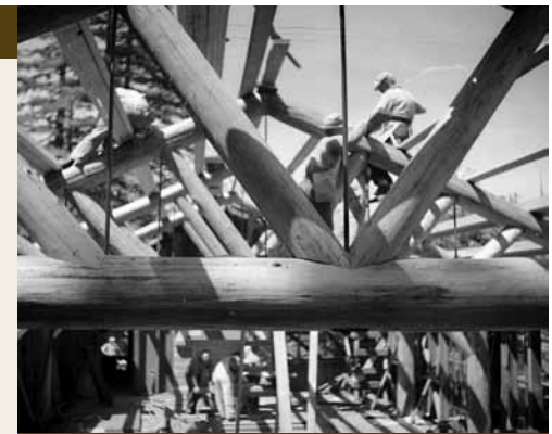
WPA crewmen working on recreation hall roof, ca. 1938
