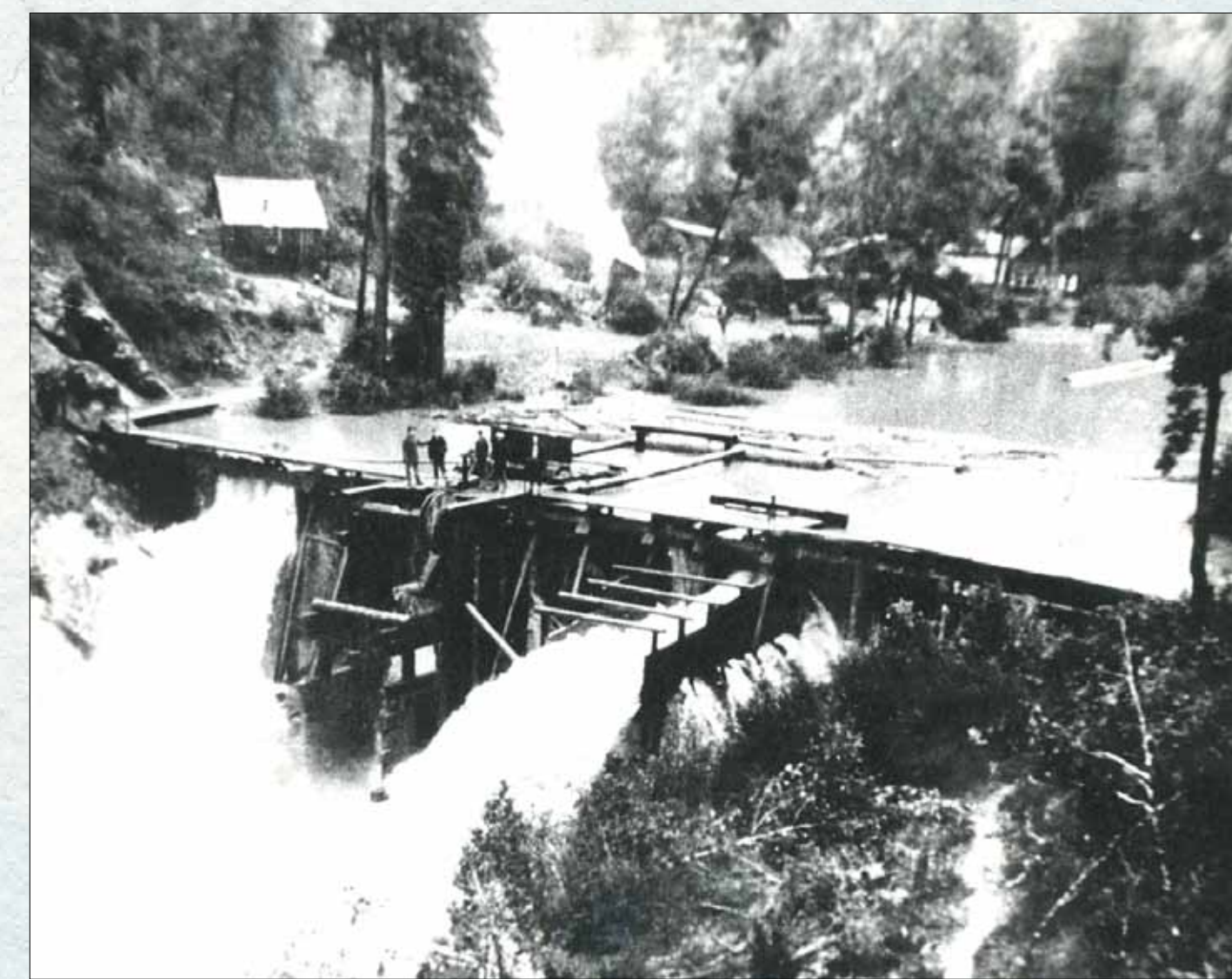
Hellsgate Dam, 35 miles upstream from New Boom, circa 1912.
