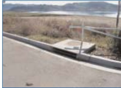
Launch ramp filtration, Lake Casitas PHOTO: Carole Iles.
