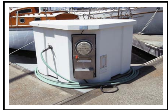
Storage Box with Anti-Siphon Hose Bibb
