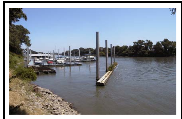
Upstream Debris Deflection Boom
