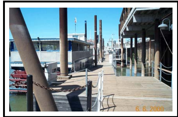
Steel Guide Piles in a River Marina
