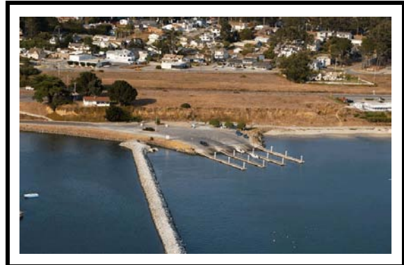
Boat Launching Facility Within Marina Basin
