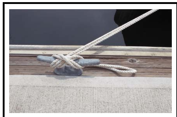
Fingerfloat Cleat Attached to Inside Waler
