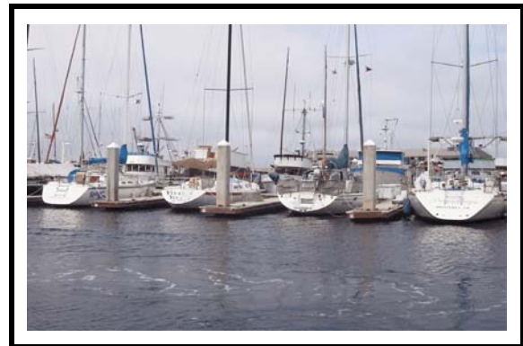
Fingerfloat Piles Adjacent to Channel
