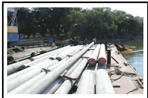
Round Concrete Piles on a Barge
