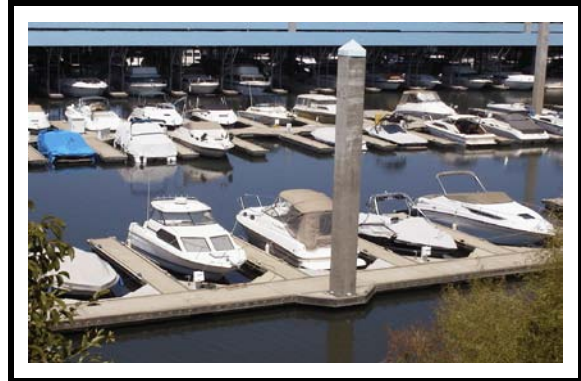
Square Concrete Guide Pile in River Marina
