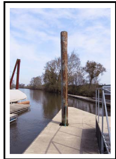
Pressure Treated Wood Pile
