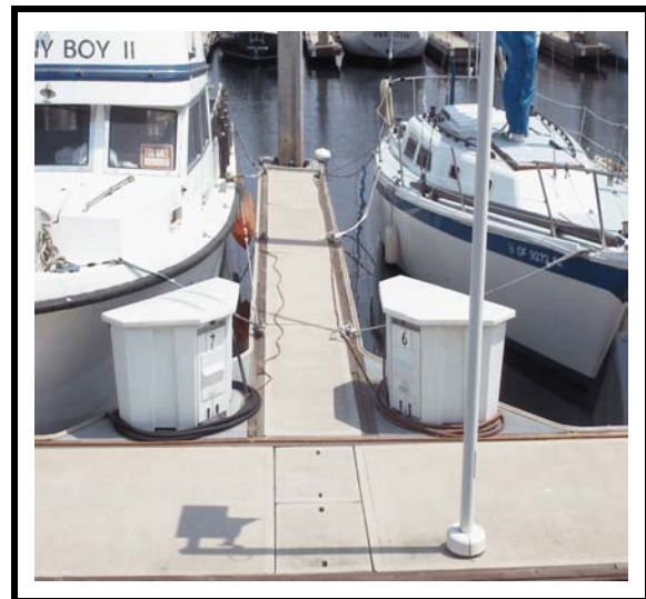
View of Fingerfloat Clear Width Including Walers
