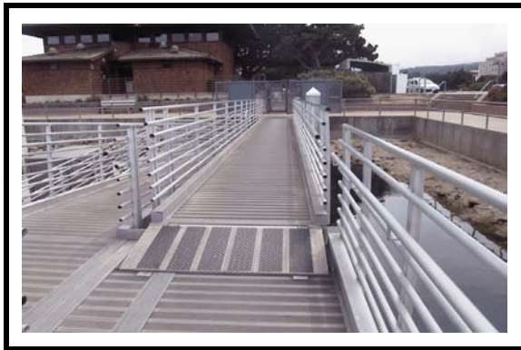
Handrails on Both Sides of a Gangway
