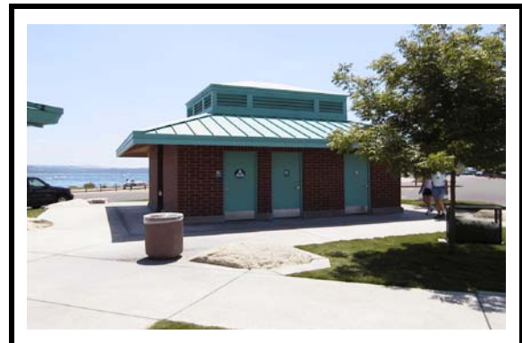
Unisex Toilet Compartment Restroom
