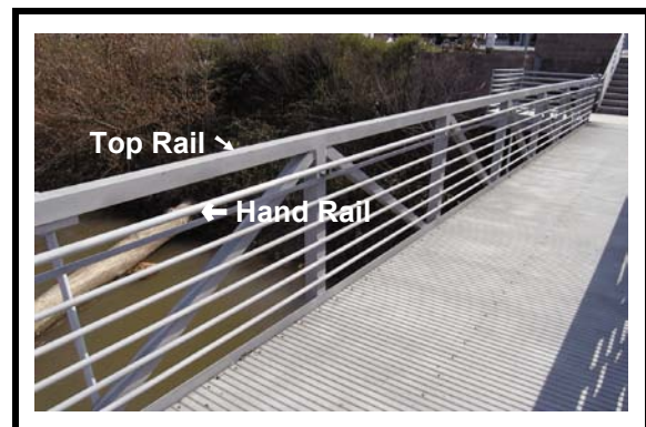
Guard Rail w/Hand Rail Meets 4" Sphere Test
