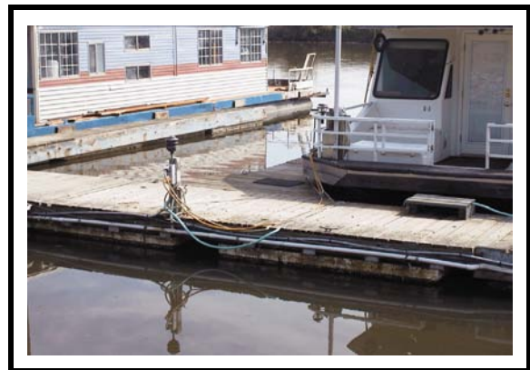
Utility Lines in Walkway Deck Gaps
