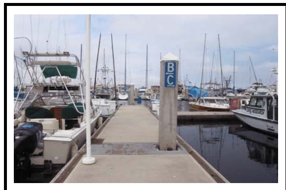
Pile Cap and Marker Signs
