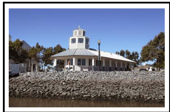
Marina Restroom Facility
