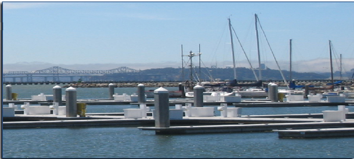
After: Newly completed ADA-compliant docks at Berkeley Marina
