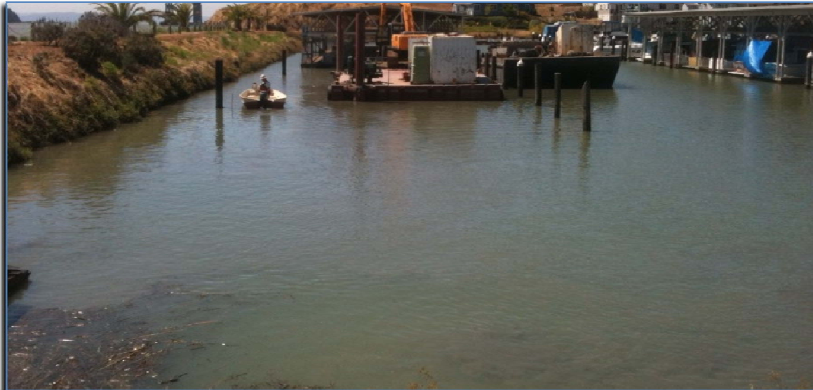
Harbor and marina slips being dredged at Glen Cove Marina
