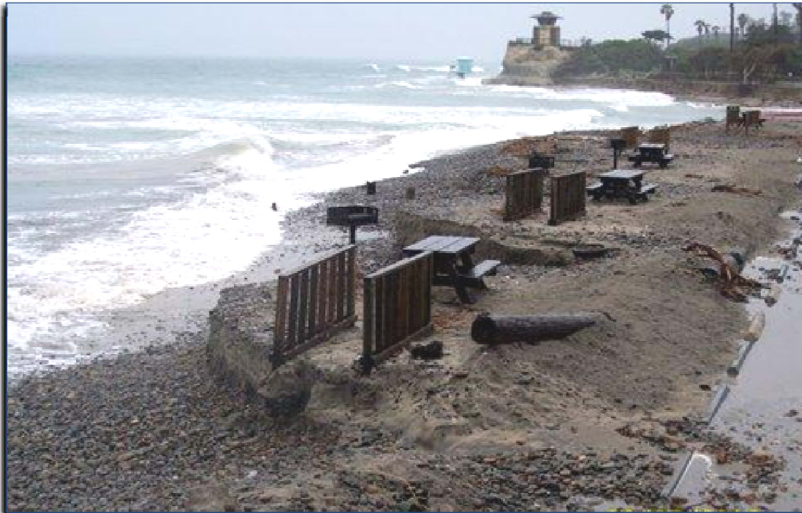
Beach erosion in early 2010 at Cardiff State Beach
