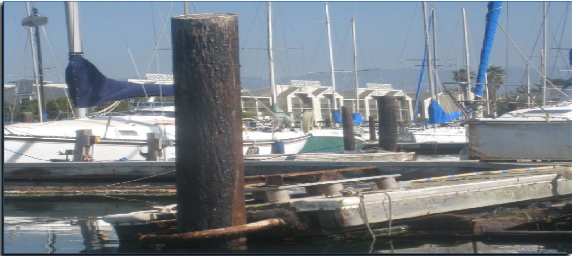
Before: Docks at Berkley Marina that are worn down and do not meet ADA standards
