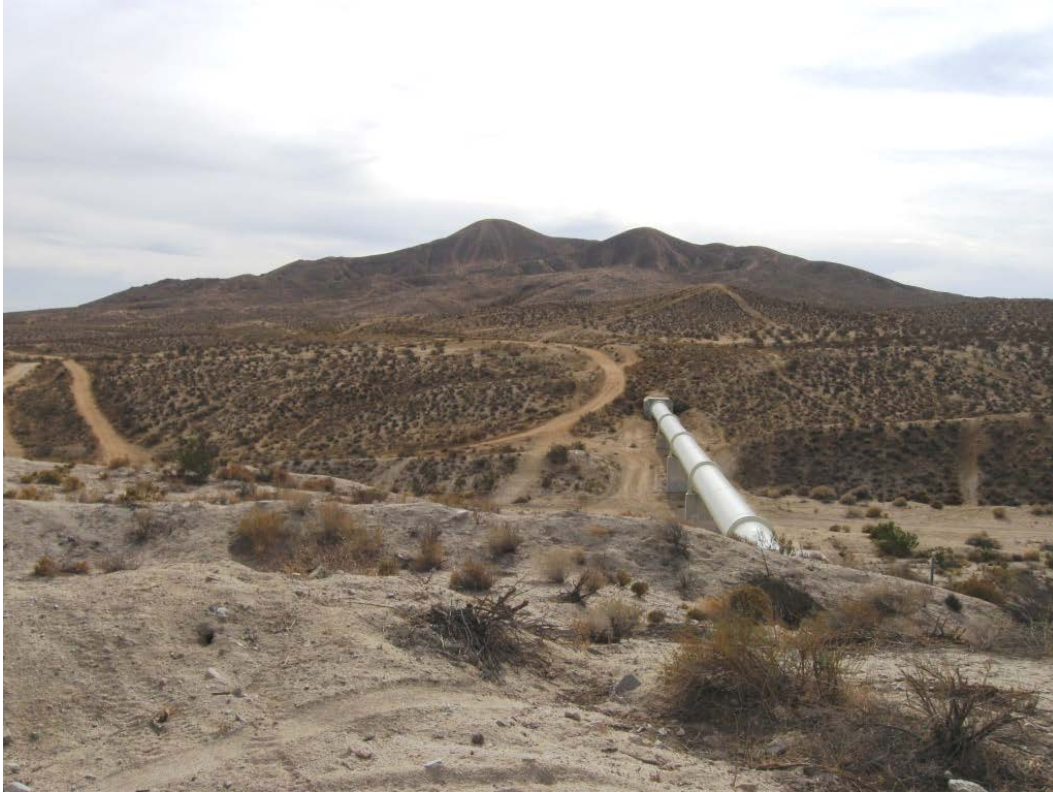
Photo 2-1. LAWPA Aqueduct Pipeline
