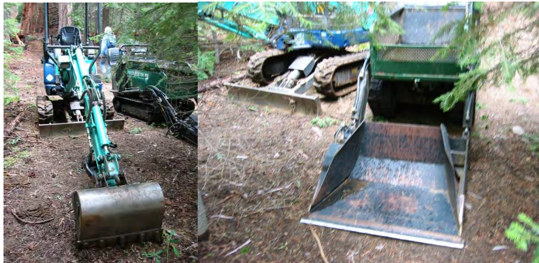
Equipment used to “maintain” the Freeman Creek Trail.
