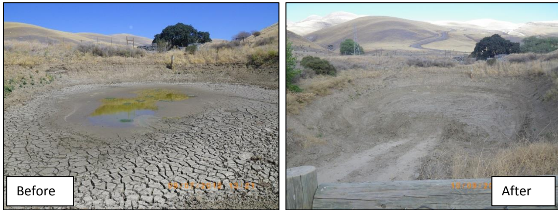
Figure 14. Tyson Basin Cleanout.
