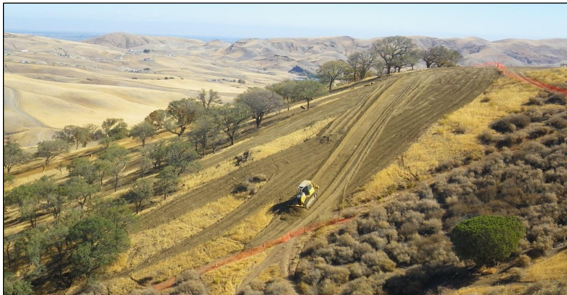
Figure 15. Sediment Reuse. The sediment from the basins is used for rehabilitation projects in the park. The photo shows Zone 47 being rehabbed.
