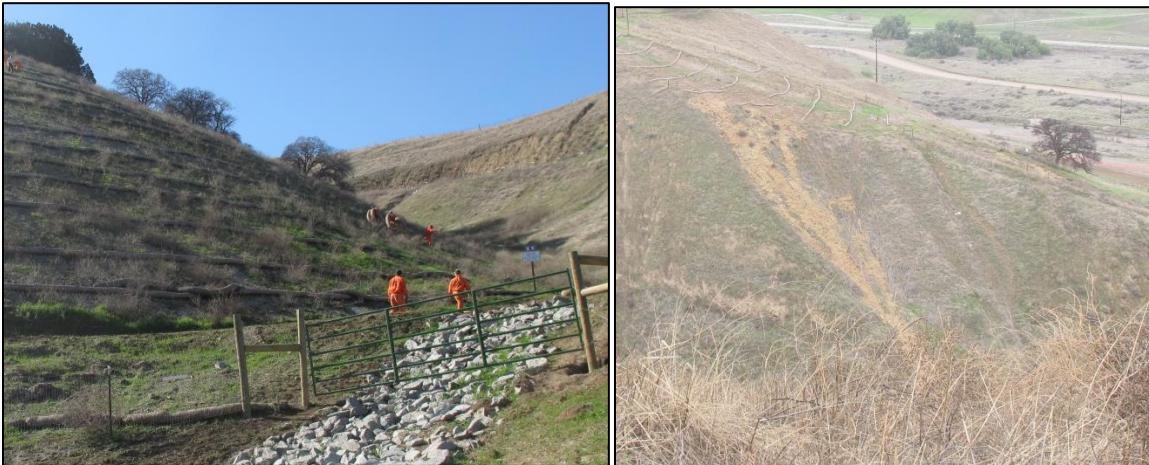
Figure 5. Off-trail Riding Correction Measure. Inmate crews are often used to implement corrective measures. Hay is typically spread over the exposed soils to reduce raindrop erosion and also to communicate to visitors that the created trail is not sanctioned.
