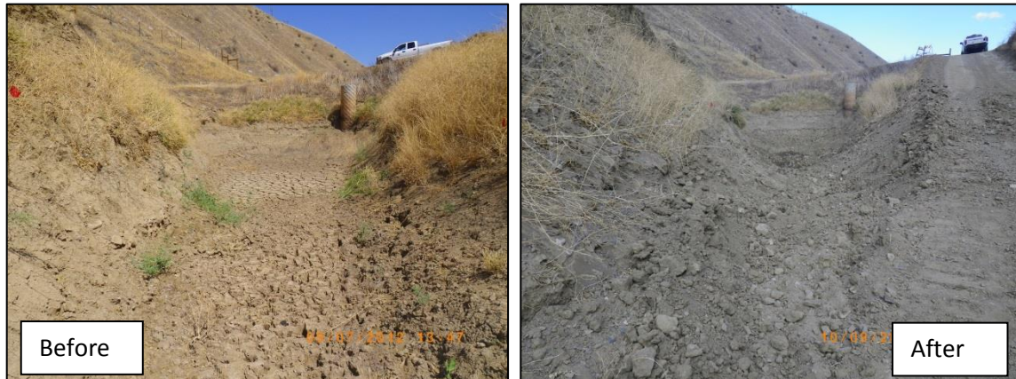
Figure 12. Kiln Basin Cleanout.
