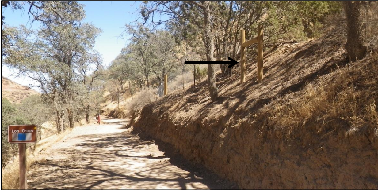
Figure 7. The Black Bear Sub-RMA. The perimeter fence (2500') was installed in order to close the area for the rehabilitation work scheduled for the next reporting cycle.
