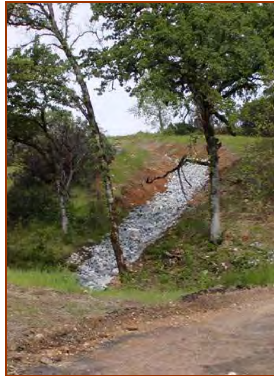
This gully could not be dewatered. It was re-graded and filled with rock, leaving sufficient cross sectional area for high discharges. (J. McCullah, 2003)
