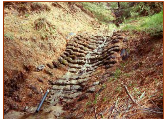
Headcut structures take runoff safely from high potential to low potential areas.
