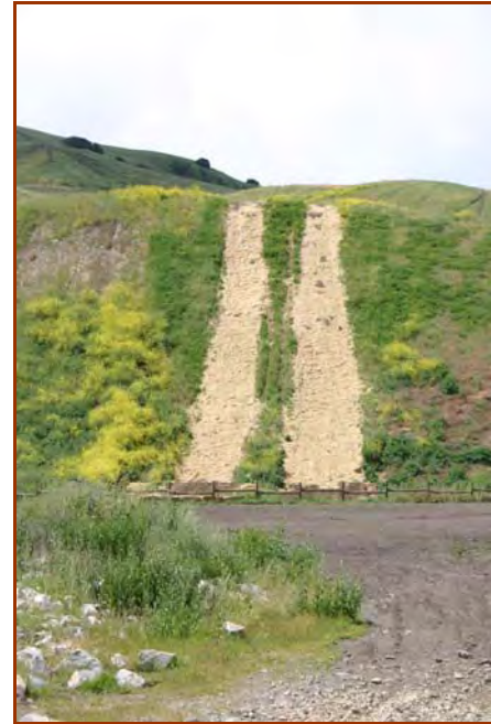
SS-5 Straw Mulching BMP used to rehabilitate a hill climb at Carnegie SVRA.
