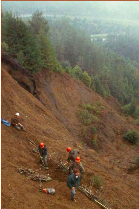
This landslide and gully repair, high above the Eel River, relied on modified Live Gully Fill Repair techniques. (J. McCullah, 2002)
