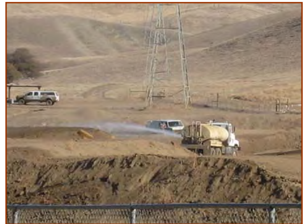
Water spraying is a temporary mechanical method that confines and settles the dust from the air by dust and water particle adhesion. (Carnegie SVRA)
