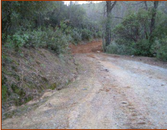
This section of a rehabilitated low-volume road is insloped. At the climbing turn in the background, the road transitions to outslope.
