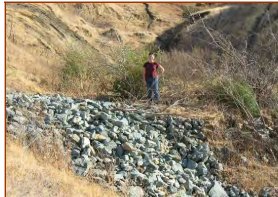
Check dams installed at Carnegie SVRA have successfully arrested gully growth for nearly 20 years.
