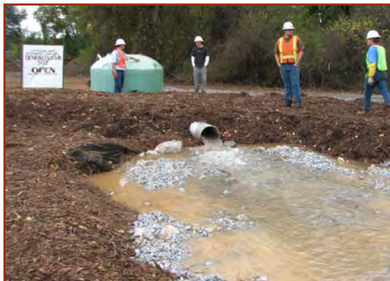
Outlet structure is non-eroding at 1/2 pipe-full discharge, approximately 10-12 fps.
