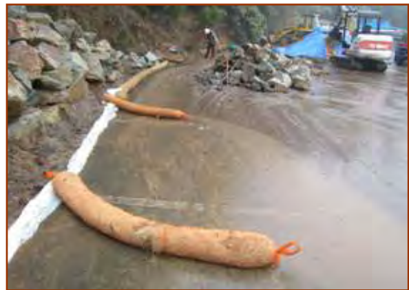
Weighted fiber rolls can be used on pavement or other surfaces where staking is not feasible.
