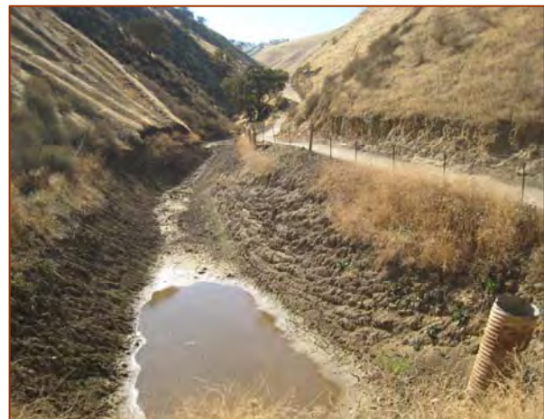
This sediment pond at Carnegie SVRA will be redesigned (2007 photo).
