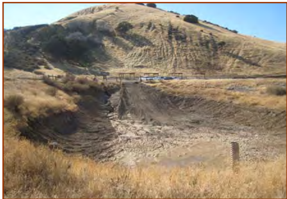
Sediment pond at Carnegie SVRA. The sediment from the prior winter was removed.
