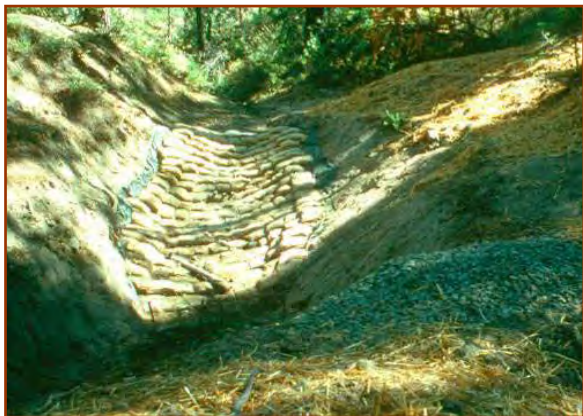
Headcut structure made from soil/cement sandbags structures.
