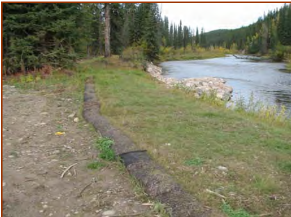
Compost blankets at vane 1 after one year. Not only did the compost blankets prevent erosion, but also helped establish native grasses. (2006)
