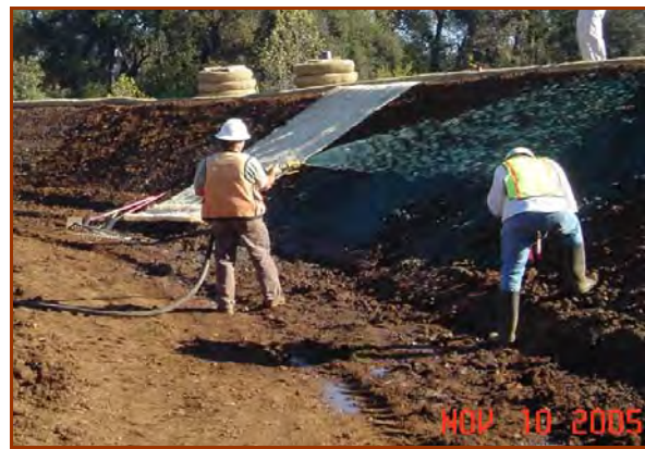
PFM (PAM Fiber Matrix) is a PAM and wood fiber mixture applied here to a slope during BMP testing at Shasta College (2005).
