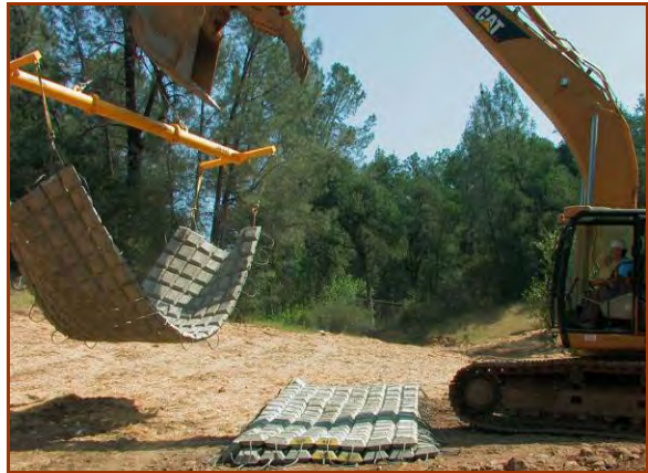
Some ACB systems are pre-cabled for installation with a spreader bar and a large excavator.
