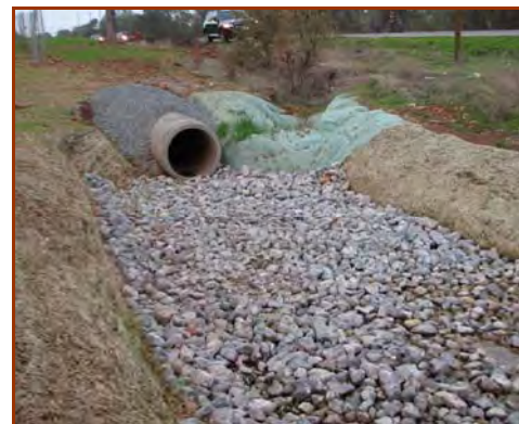
Riprap apron-type Energy Dissipator.
