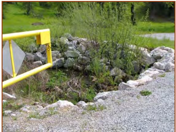
Photo series showing installation of Vegetated Riprap with Bent Poles.
