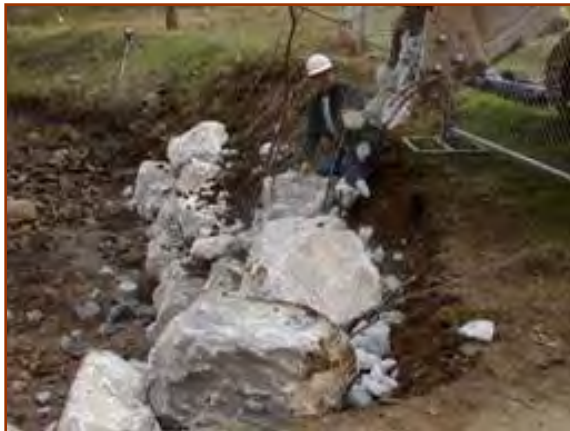
Photo series showing installation of Vegetated Riprap with Bent Poles.
