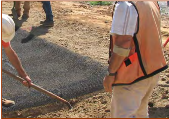
A 3-dimensional nylon TRM is being keyed into a terminal check slot.
