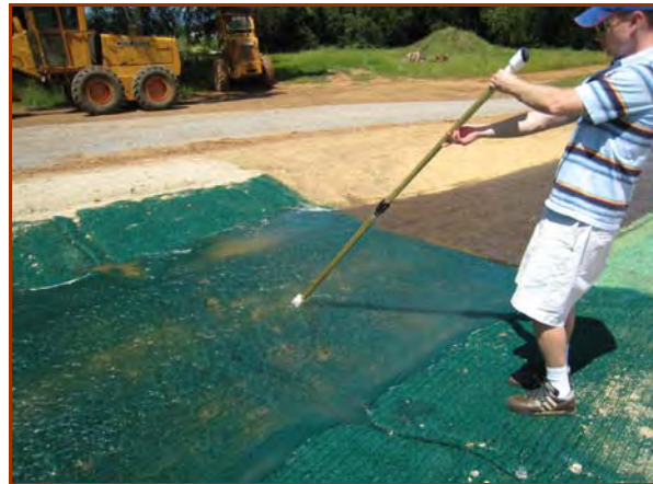
Hydrologists measured 4 ft/sec over the un-vegetated polypropylene mat with no erosion.
