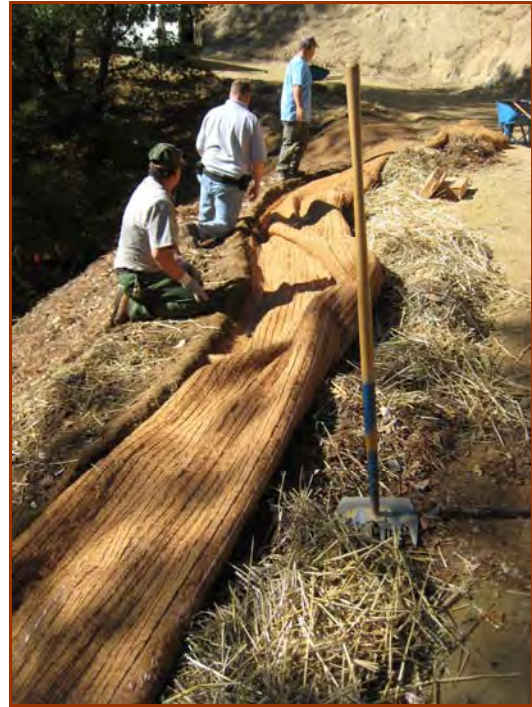
Anchor ECBs in a trench at top of slope.
