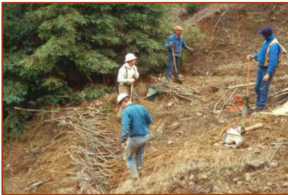
Another technique used was Modified Brush Layers , a variation on Live Gully Fill.
