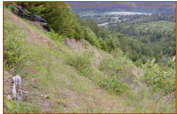
After only two winters, the gullies and landslide scars are revegetating well. Native grasses were also used. (J. McCullah, 2004)
