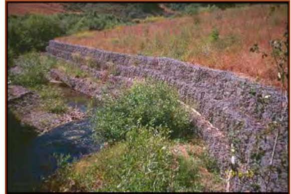
July 2000. After the first winter the scour mattress “dropped” into place as designed and a few willow stakes successfully established.
