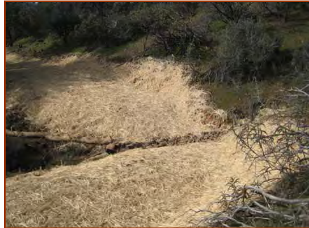
Terrain dips are spaced according to the natural topography, and located where the trail or road cutslope decreases (or disappears). This terrain dip is also armored with rock found on-site.
