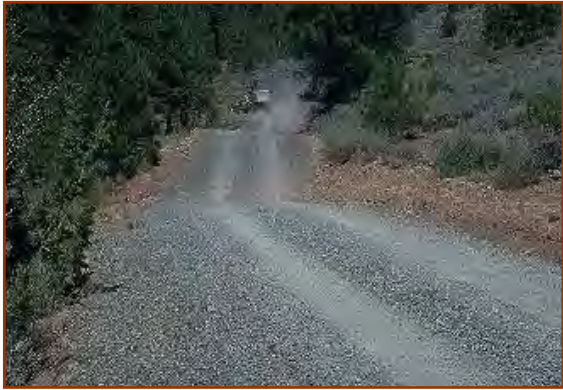
Outsloped roads and trails used in combination with dips can reduce maintenance costs, decrease soil erosion, and reduce sediment delivery and loading (sedimentation) to downstream resources.
