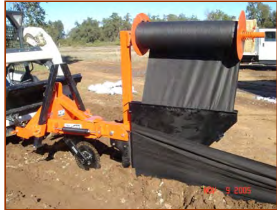
Silt fence installed by slicing method.
