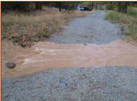
Armored crossings can withstand high velocities without eroding. (J. McCullah photo, 2007)
