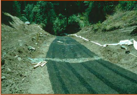
This gully was filled, re-graded, and lined with soil-filled and vegetated TRM, designed for the 10-yr RI storm. (J. McCullah, 1992)
