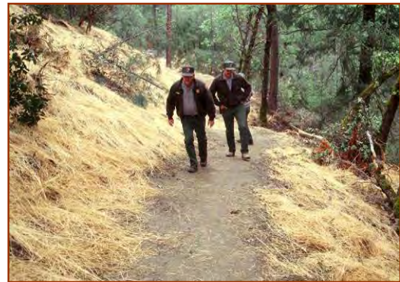
The same trail section after outslipping.
