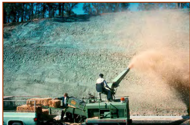
Straw blower used for mulch application on steep slope.
