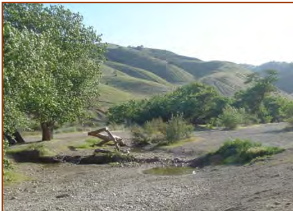
Rock-filled gabion basket “check dams” failed after 15+ years in Corral Hollow Creek, Carnegie SVRA.
