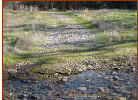
The temporary crossing shown above has geotextile underlying clean, angular aggregate.
