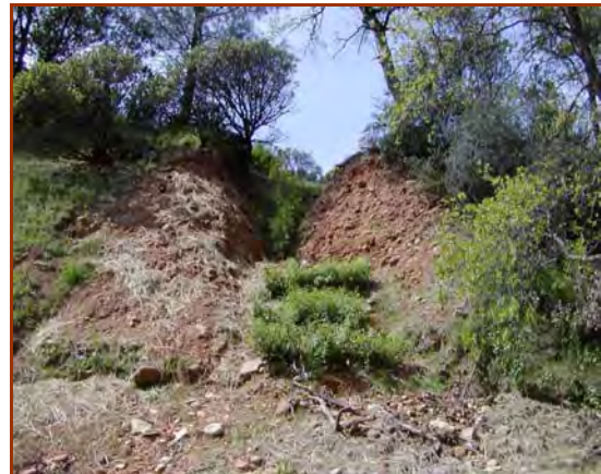
This gully was dewatered and treated with a Live Pole Drain and Modified Brush Layers. (J. McCullah, 2003)
