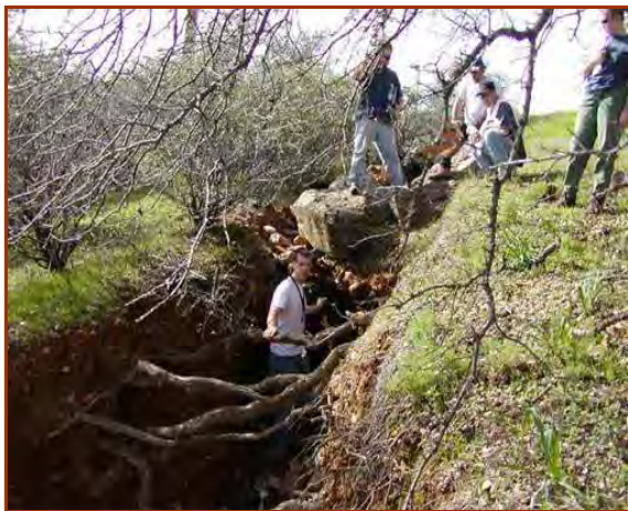
This gully could not be dewatered. It was re-graded and filled with rock, leaving sufficient cross sectional area for high discharges. (J. McCullah, 2003)
