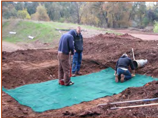
Riprap apron installed step by step. First the apron area, determined by culvert size, e.g., 4.5 \times \text{Dia} = \text{apron length} .
