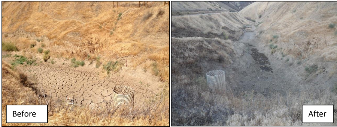
Figure 14. Kiln Basin Cleanout.
