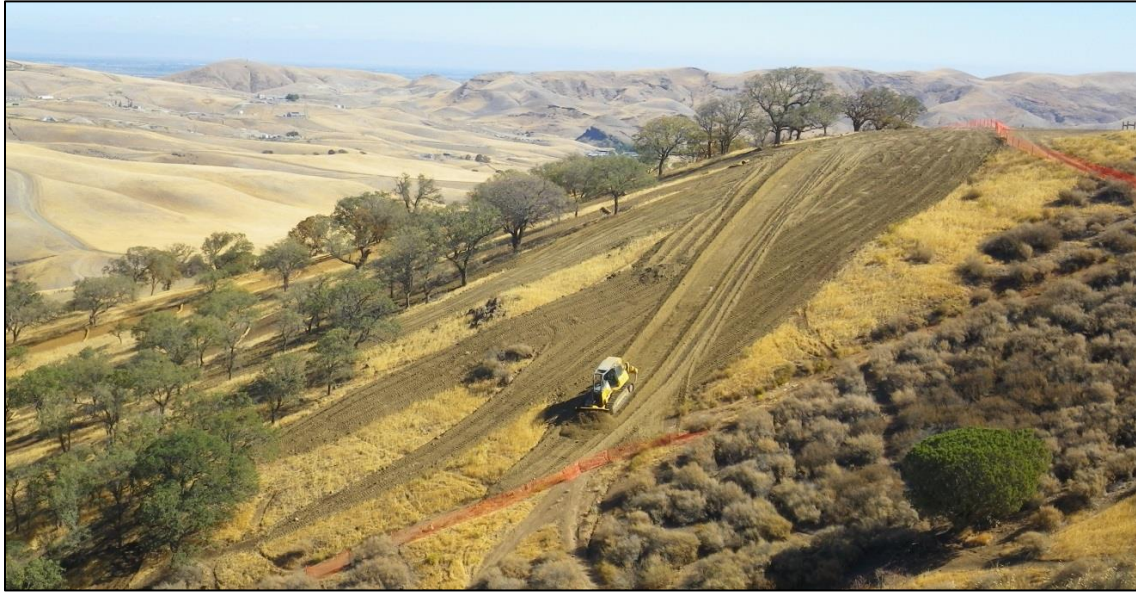
Figure 17. Sediment Reuse. The sediment from the basins is used for rehabilitation projects in the park. The photo shows Zone 47 being rehabbed.
