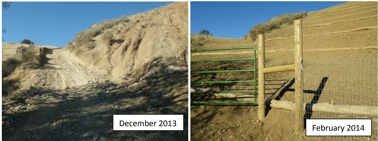
Figure 8. Rehabilitation of Through Cut. Area was closed to eliminate off-trail riding, brought up to grade, and restored.
