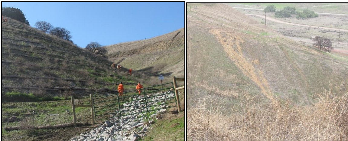
Figure 5. Off-trail Riding Correction Measure. Inmate crews are often used to implement corrective measures. Hay is typically spread over the exposed soils to reduce raindrop erosion and also to communicate to visitors that the created trail is not sanctioned.
