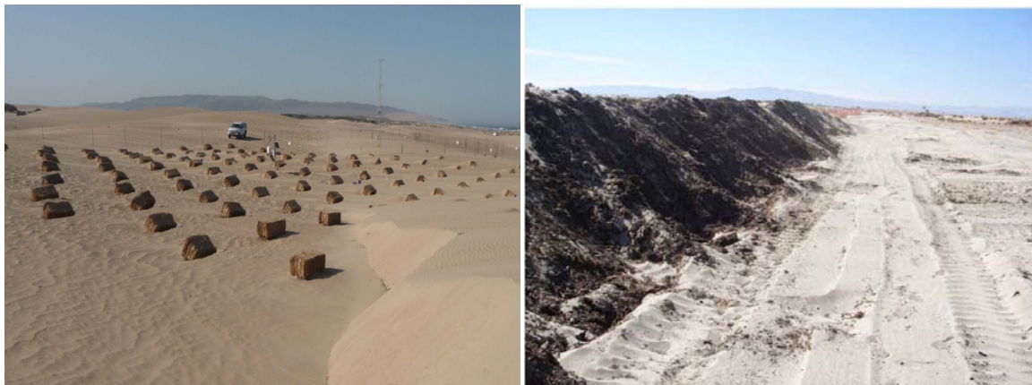
Figure 2-12 Artificial Roughness Dust Control Measures. Left: Straw bales at Oceano Dunes SVRA. Right: Wood chip berm at Owens Lake (Image Source: Farber et al. 2010).
