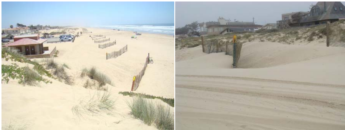
Figure 2-13 Wind fencing at Pier Avenue and Strand Way. Left: Wind fencing at Pier Avenue and Strand Way; Right: Sand accumulation at wind fence on Strand Way.
