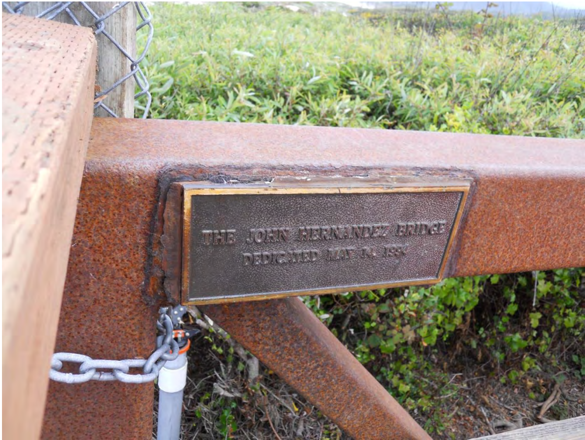
Bridge Dedication Plaque
