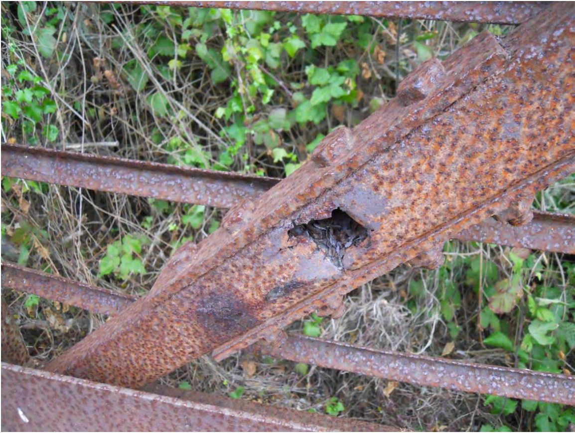
Truss Midspan Diagonal Splice – Span 3
