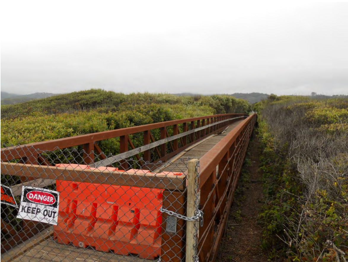
Truss Span looking East
