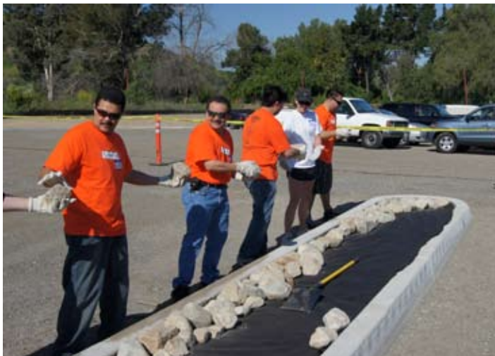
Volunteers and staff fill parking lot islands with new river rock at Chino Hills SP.
