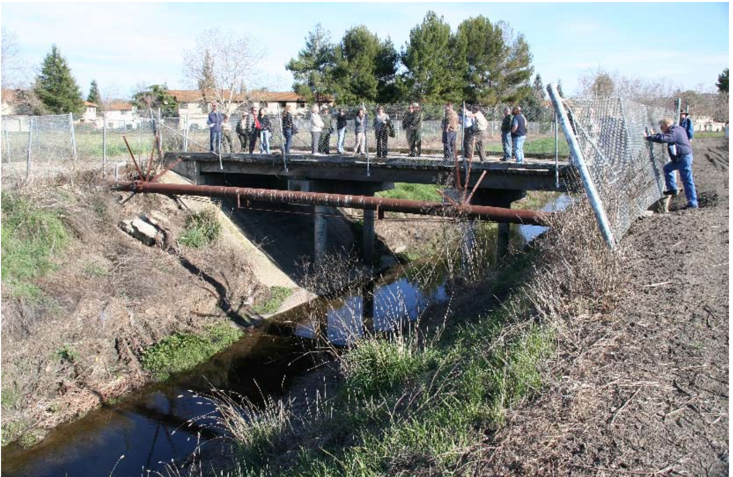
San Jose - On the tour of the property, the group stopped at a bridge across Canoas Creek, which will be changed from a ditch back to a natural, flowing creek and seasonal wetland area that will provide for increased wildlife in the area and the opportunity for interpretation and education programs for school groups and others.
