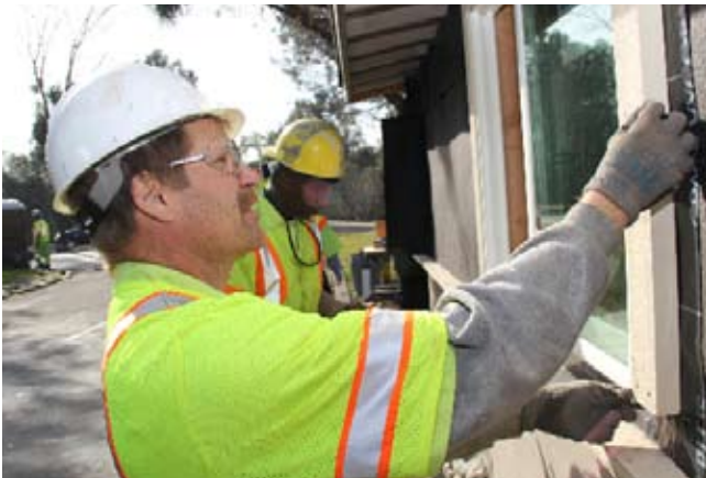
A CalPIA worker frames a window at the front entry kiosk.
