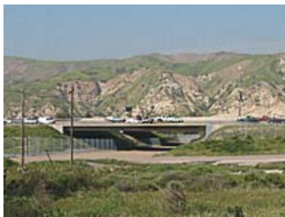
Coal Canyon wildlife linkage
