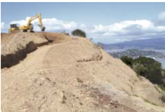
Road removal and peak restoration at Angel Island State Park
