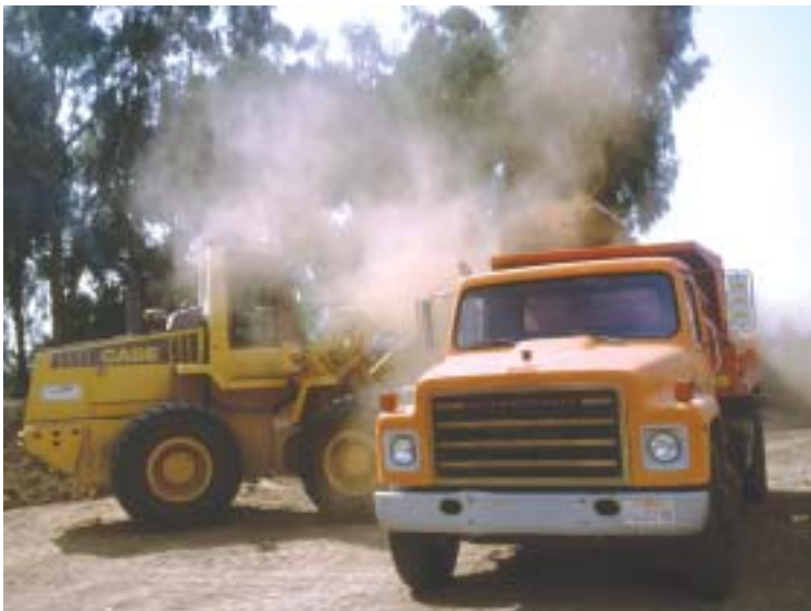
Dirt removal at Will Rogers State Historic Park
