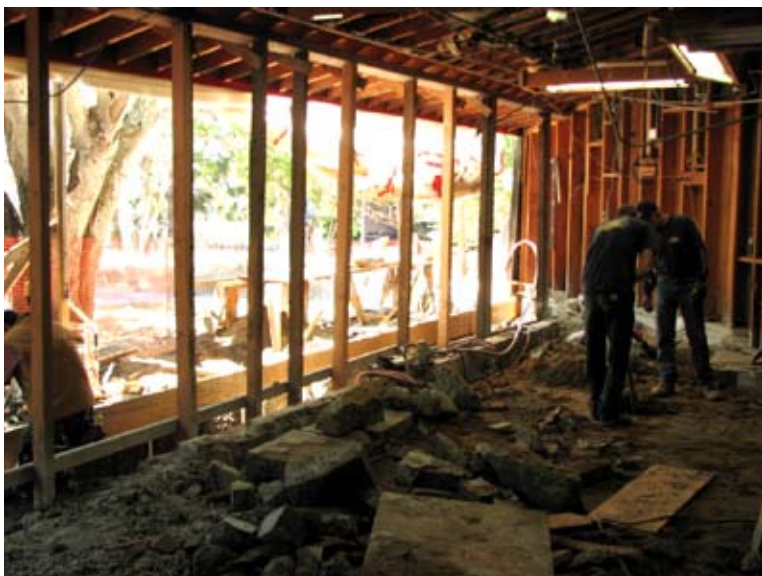
Workers demolish Training Center restrooms.
