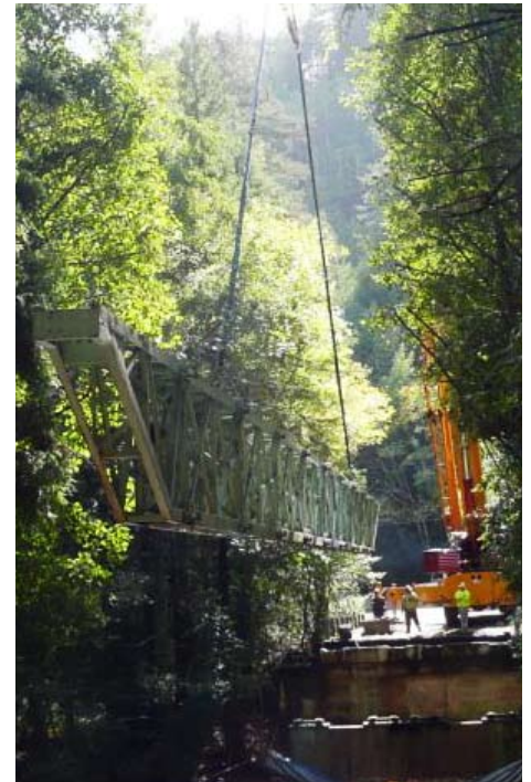
Left: The main bridge to the campground before removal. Right: A crane lifts one of the steel supports for the main bridge to the campground.
