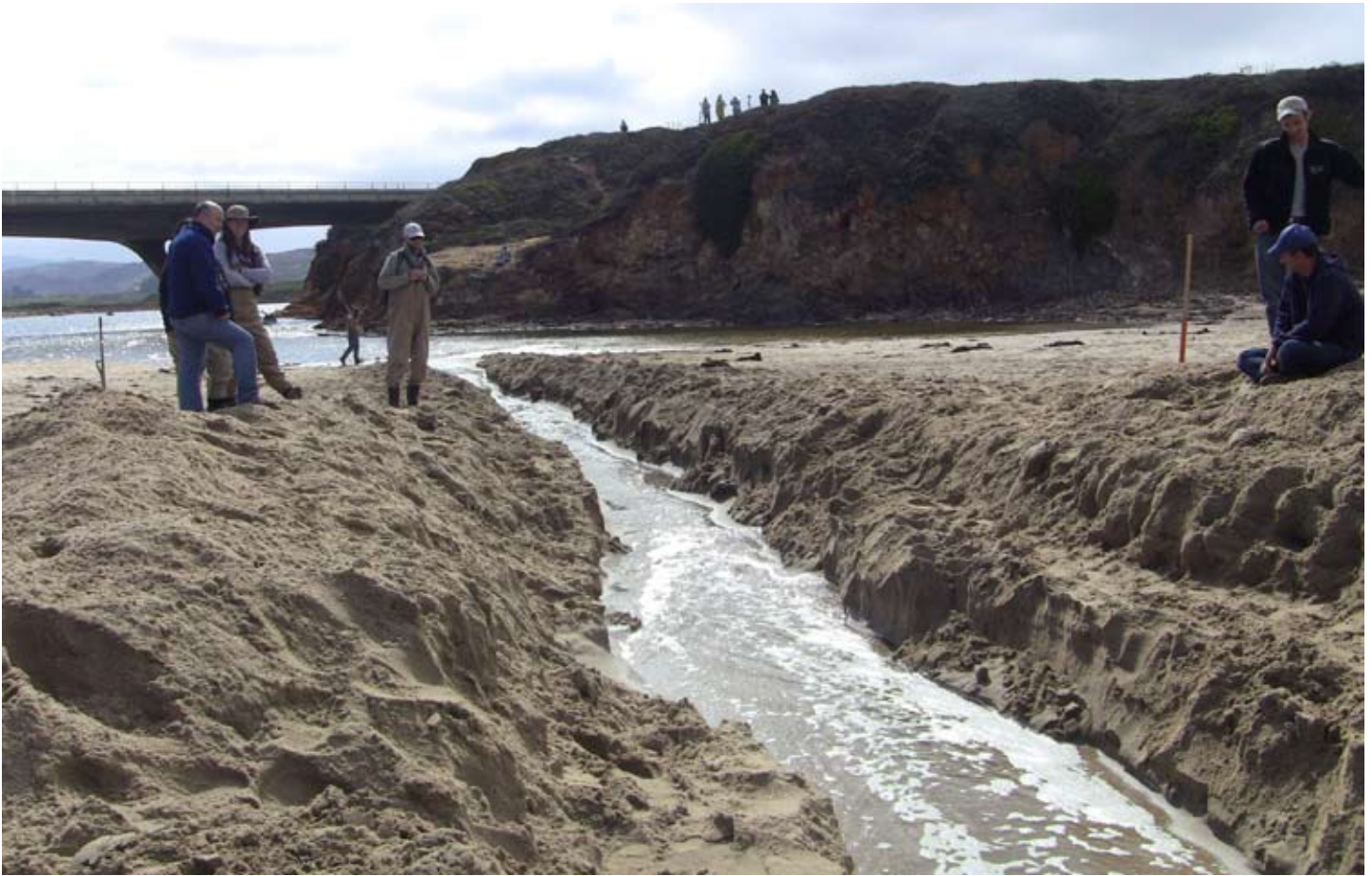
Volunteers and youth from Santa Cruz County Juvenile Hall hand-dig a breach to allow water flow between the ocean and the Pescadero Marsh. Photo by Sarah Swenty, USFWS.
