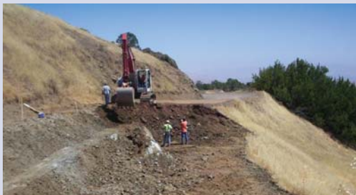
Park road construction
