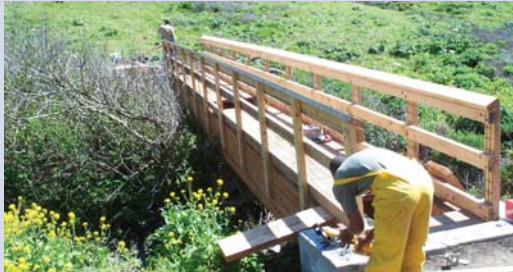
Trail bridge construction
