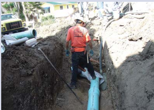
Utility construction at a state park
