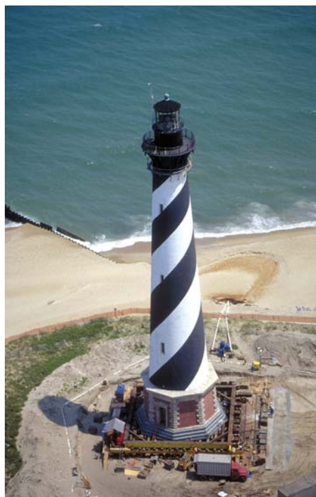
The Cape Hatteras lighthouse being prepared to be moved to keep it above the rising sea.
