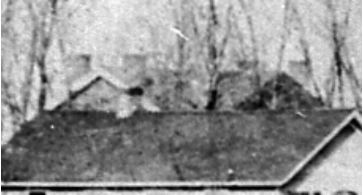
Figure 16. Detail from the 1858 Rancho Chico Buildings Overview. Courtesy of CSU, Chico, Meriam Library, Special Collections P13244.
