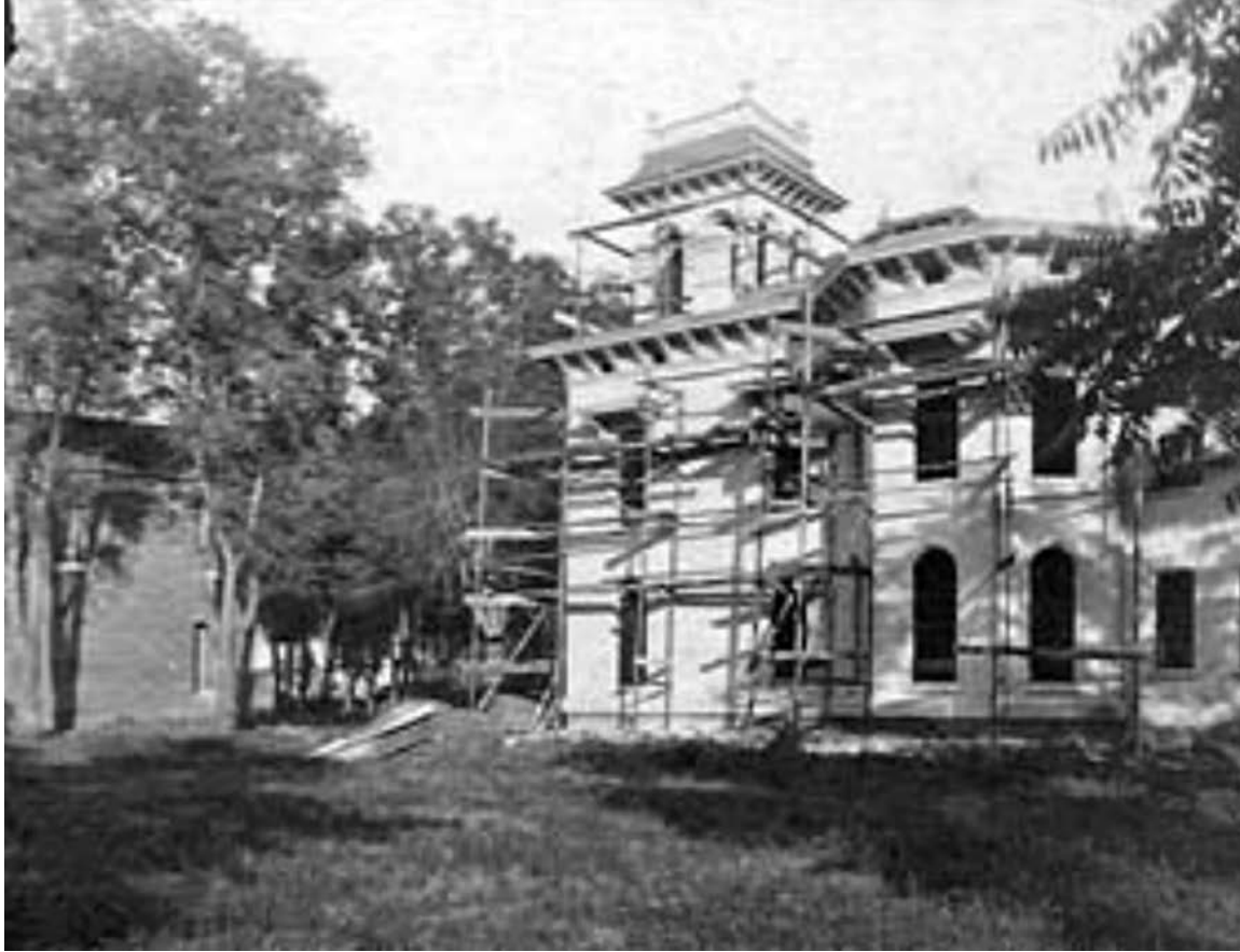
Figure 18. Bidwell Mansion under Construction circa 1866–1868 showing SW Corner of the Federal Adobe (left mid-ground).
