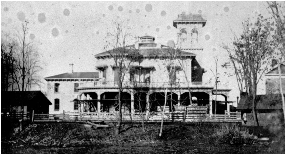
Figure 17. Bidwell Mansion under Construction circa 1866–1868 showing the Federal Adobe (right mid-ground). Courtesy of Bidwell Mansion State Historic Park, Visitor Center.
