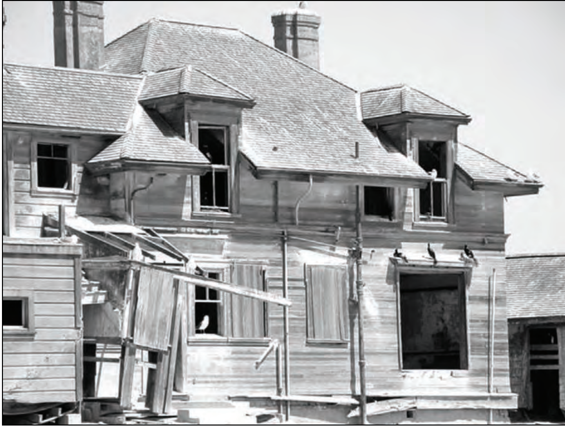
Figure 75. Keeper's Dwelling (1906 Addition), 2005.
