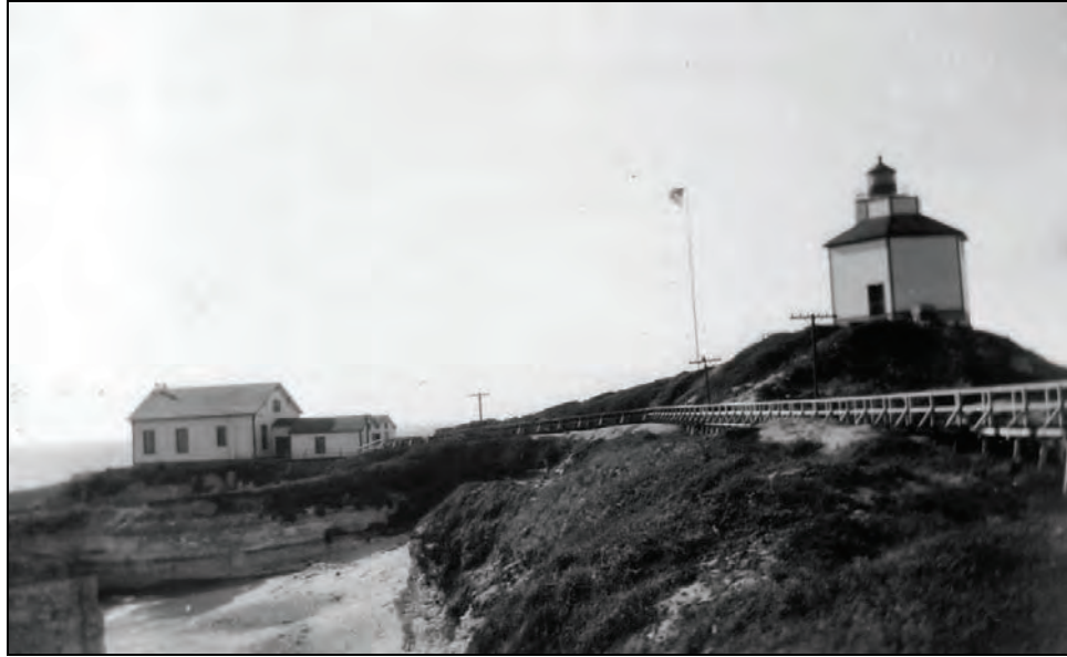
Figure 47. Wood Walkway (Catwalk) from Keeper's Dwelling to Fog Signal Building (at left), Light on Tank House, 1926.
