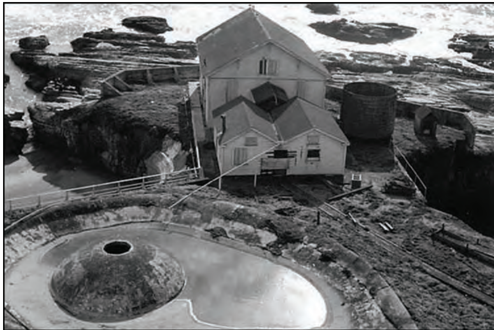
Figure 79. Fog Signal Building with Water Tank and Distillate House to the Right, 1957.
