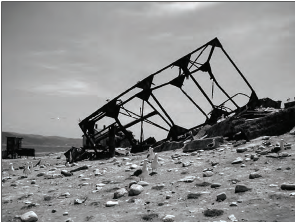
Figure 103. Steel Light Tower, 2005.
