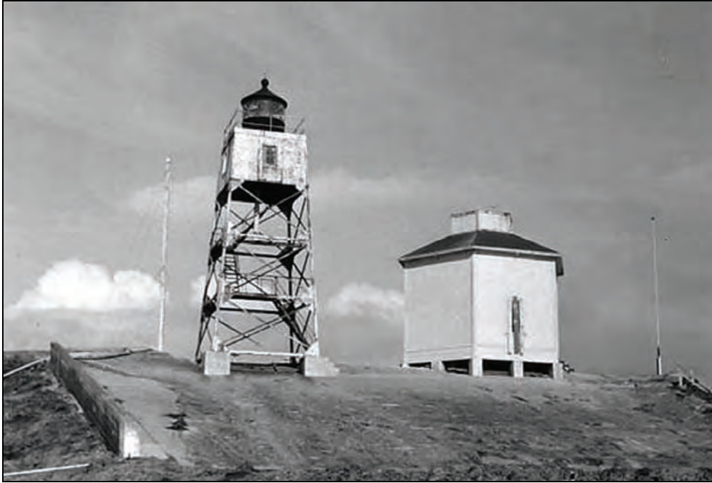
Figure 100. Steel Light Tower adjacent to Water Tank, 1957.
