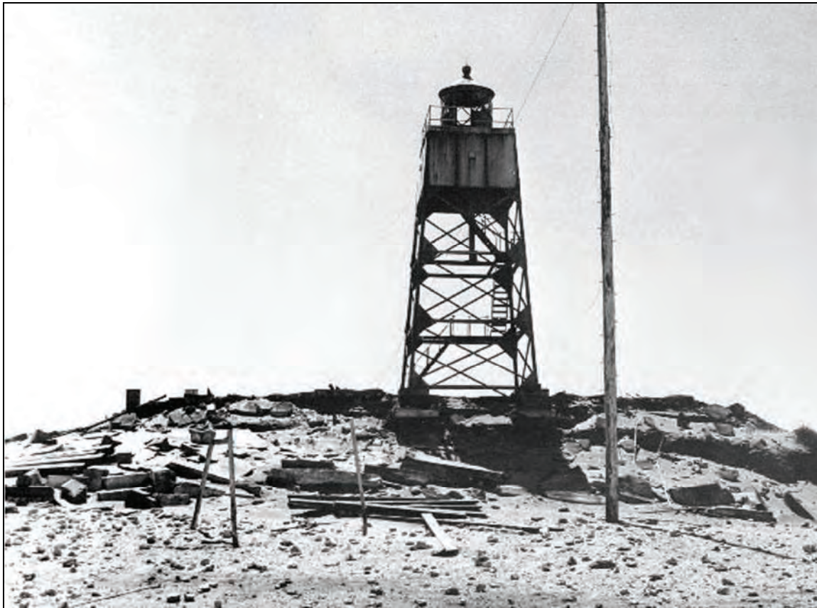
Figure 56. Steel Light Tower shortly before being cut down.
