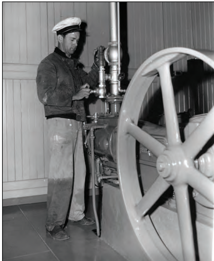
Figure 43. U.S. Coast Guardsman working on Air Compressor in Fog Signal Building, 1948.
