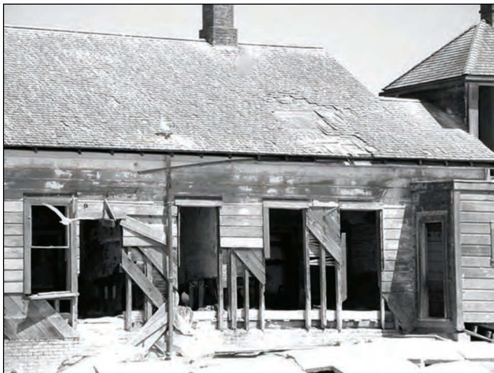
Figure 66. Keeper's Dwelling, Original Portion, West Side, 2005
