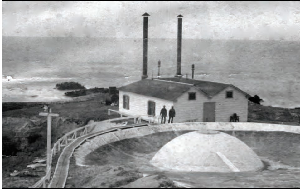
Figure 78. Second Fog Signal Building (built 1881) in front of Water Shed and Cistern, circa late 1880s.
