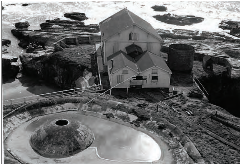
Figure 46. Fog Signal Building, 1957.
