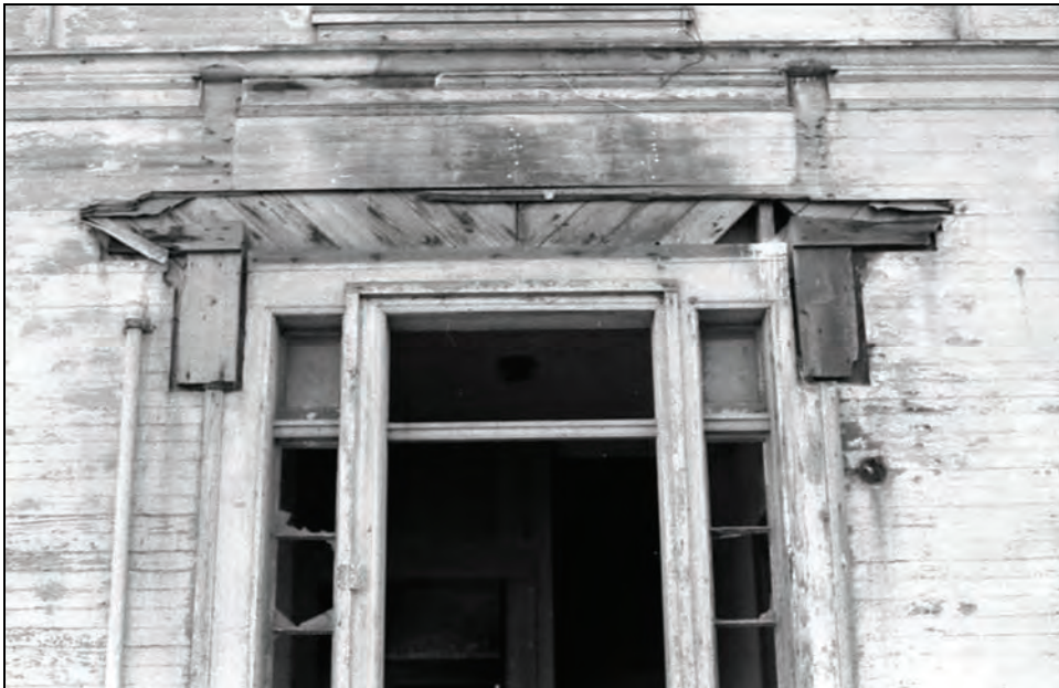
Figure 72. Front (east) Entrance to Keeper's Dwelling (1906 Addition), 1982.
