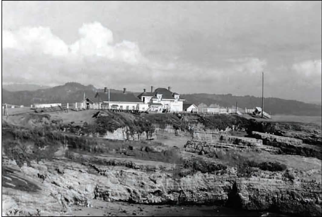
Figure 58. Keeper's Dwelling, Original on left, 1906 Addition on right, looking South, circa 1950s.
