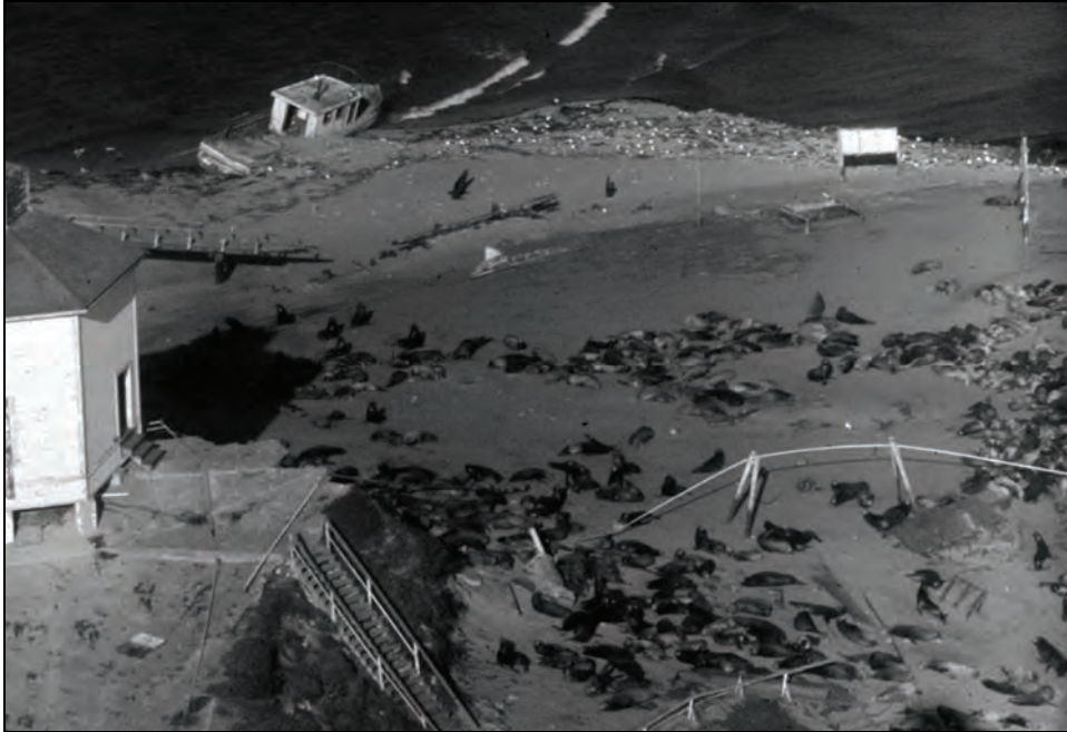
Figure 124. Portion of Water Tank Structure, circa 1961.
