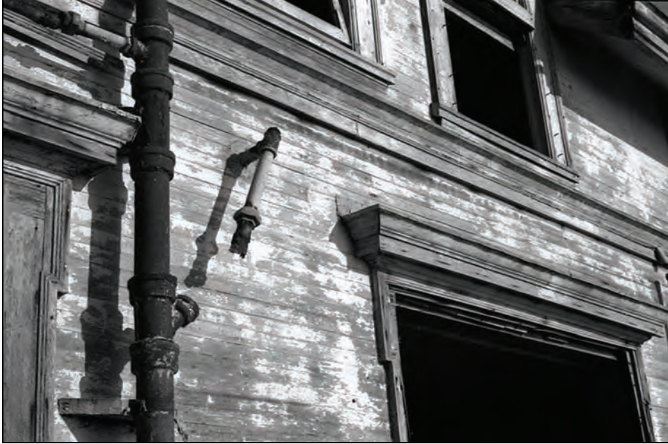
Figure 71. Exterior of West Wall, Keeper's Dwelling (1906 Addition), showing Broken Iron Pipes, Window Frames, and Molding, 1982.
