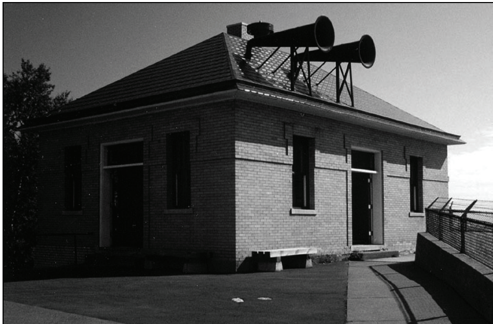
Figure 33. Fog Horn Building at Split Rock Light Station, Minnesota. Photograph by Dave Wobser.
