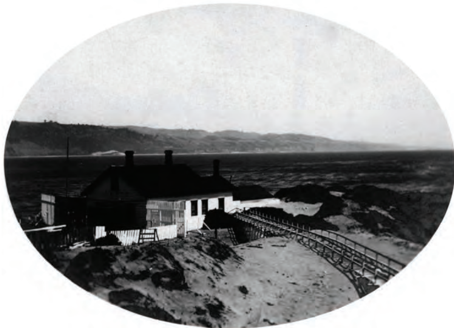
Figure 126. Fog Signal Building looking South, Unknown Date.
