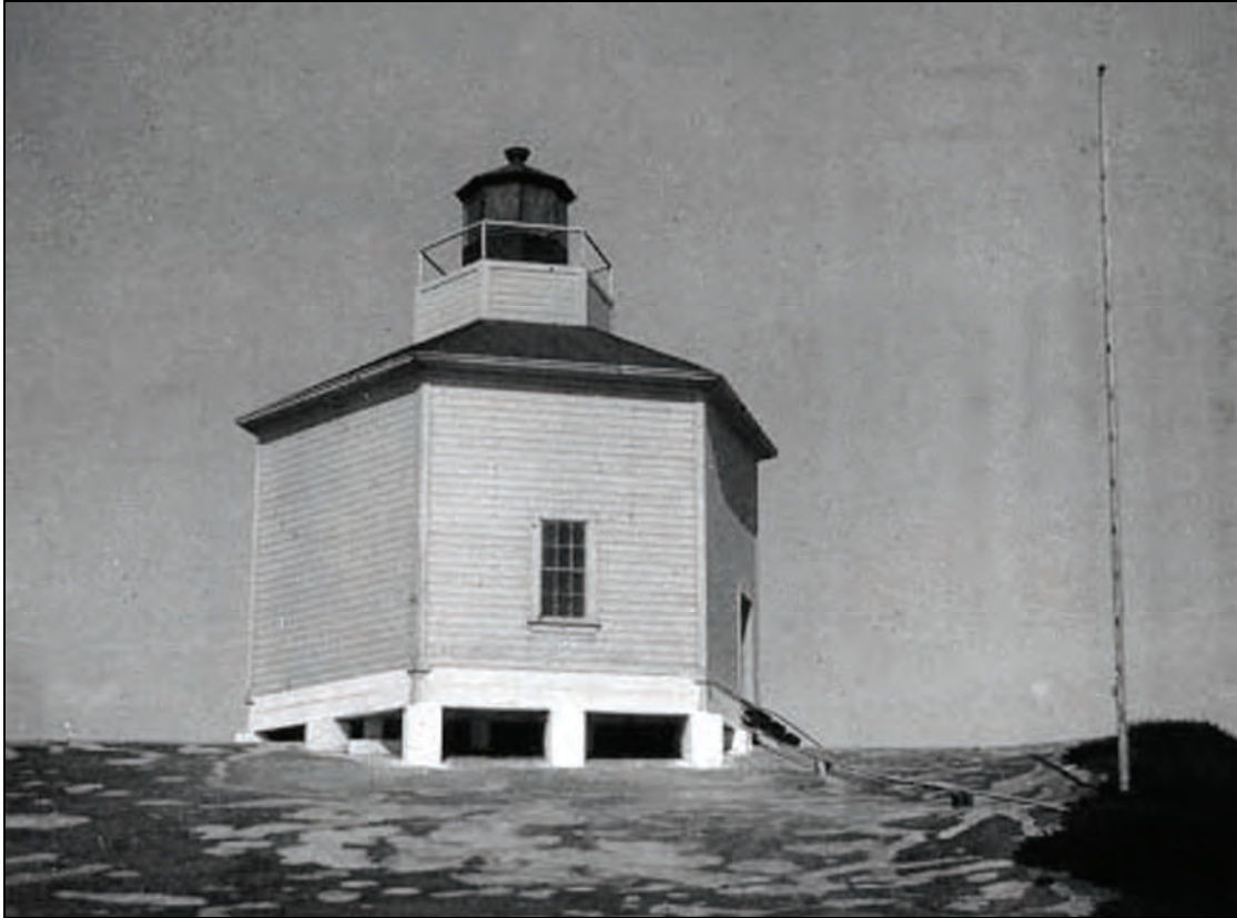
Figure 108. Tank House with Light at Top, Unknown Date.
