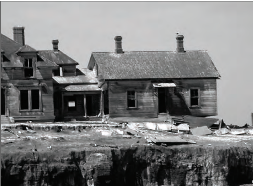
Figure 64. Keeper's Dwelling, Original on right, 1906 Addition on left, 2005.
