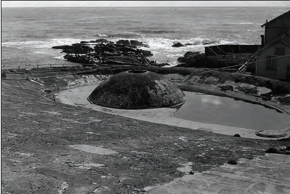
Figure 110. Cistern at the Base of the Water Shed, 1957.
