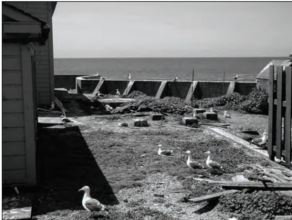
Figure 107. Foundation for Water Tank adjacent to Fog Signal Building, 2005.
