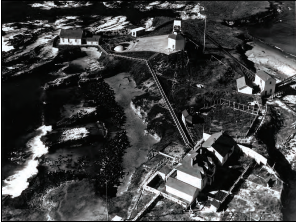
Figure 114. Overview of Island with Boat House, Coal House, and Carpenter's Shop visible at Right, 1953.
