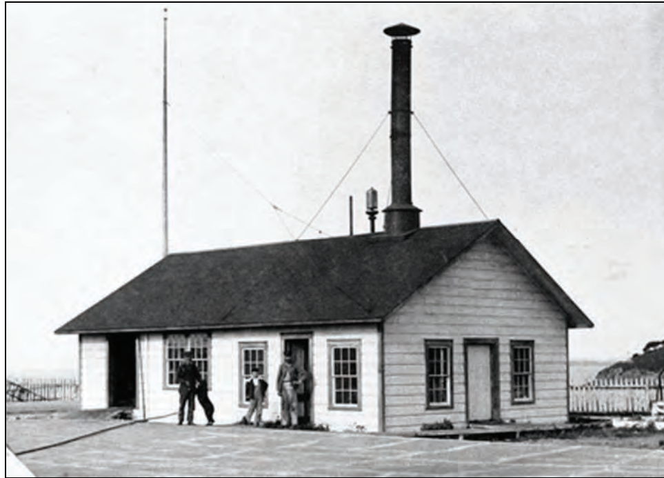
Figure 32. Fog Signal Building at East Brother Lighthouse, Richmond, California. Steam whistle is immediately left of large smokestack. Photograph by Nels Stenmark.
