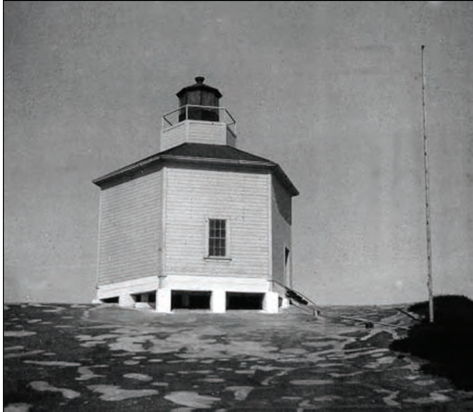
Figure 40. Tank House with Light at Top.
