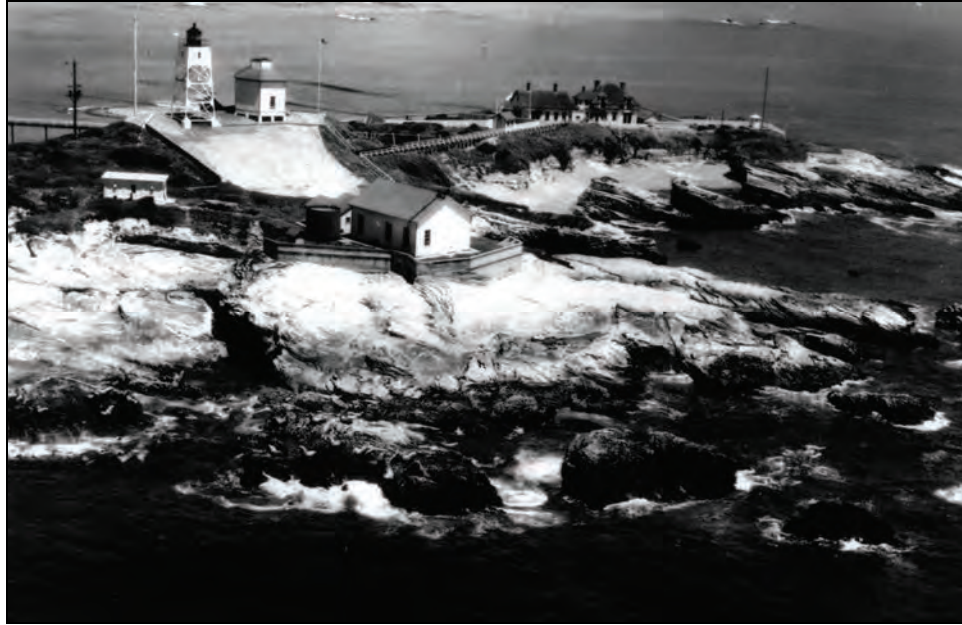
Figure 98. Overview of Light Station with Light Tower visible at Left, 1953.
