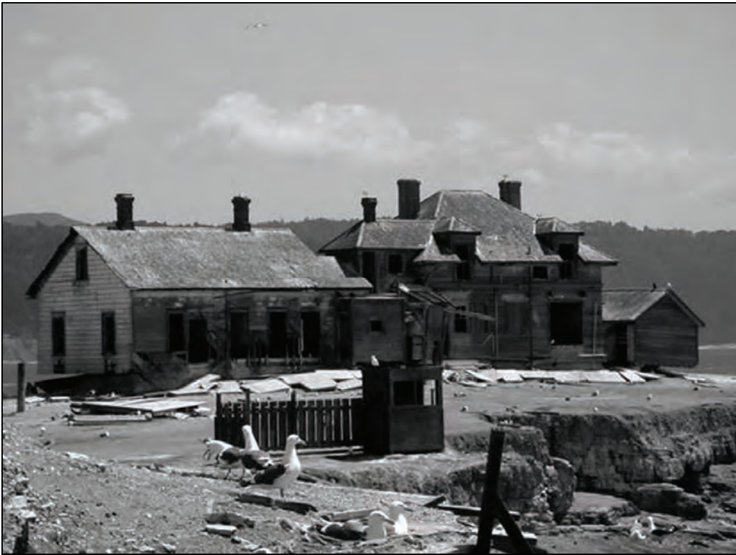
Figure 61. Keeper's Dwelling, looking Southeast, 2005.
