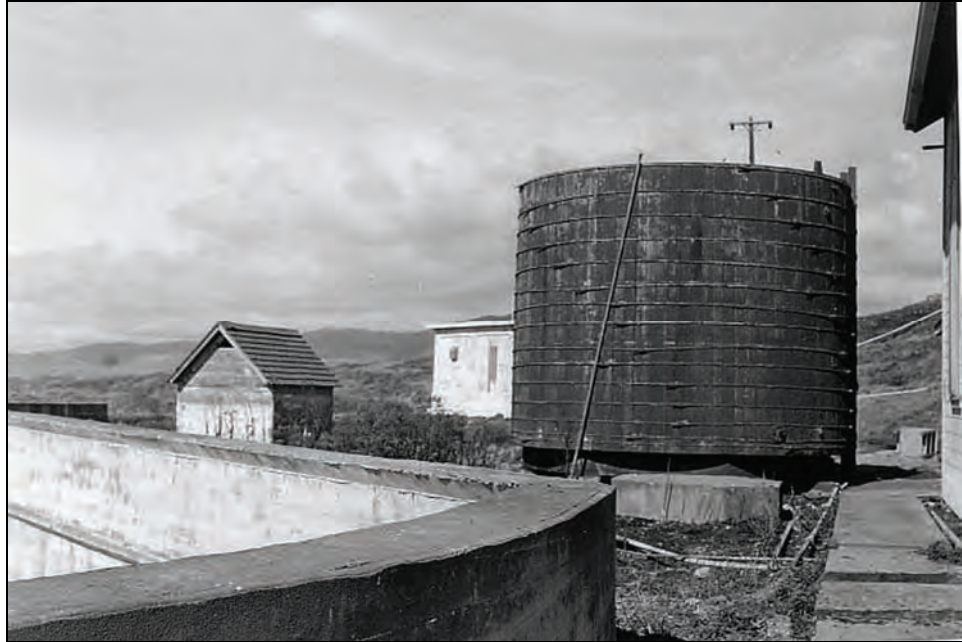
Figure 106. Water Tank adjacent to Fog Signal Building, 1957.
