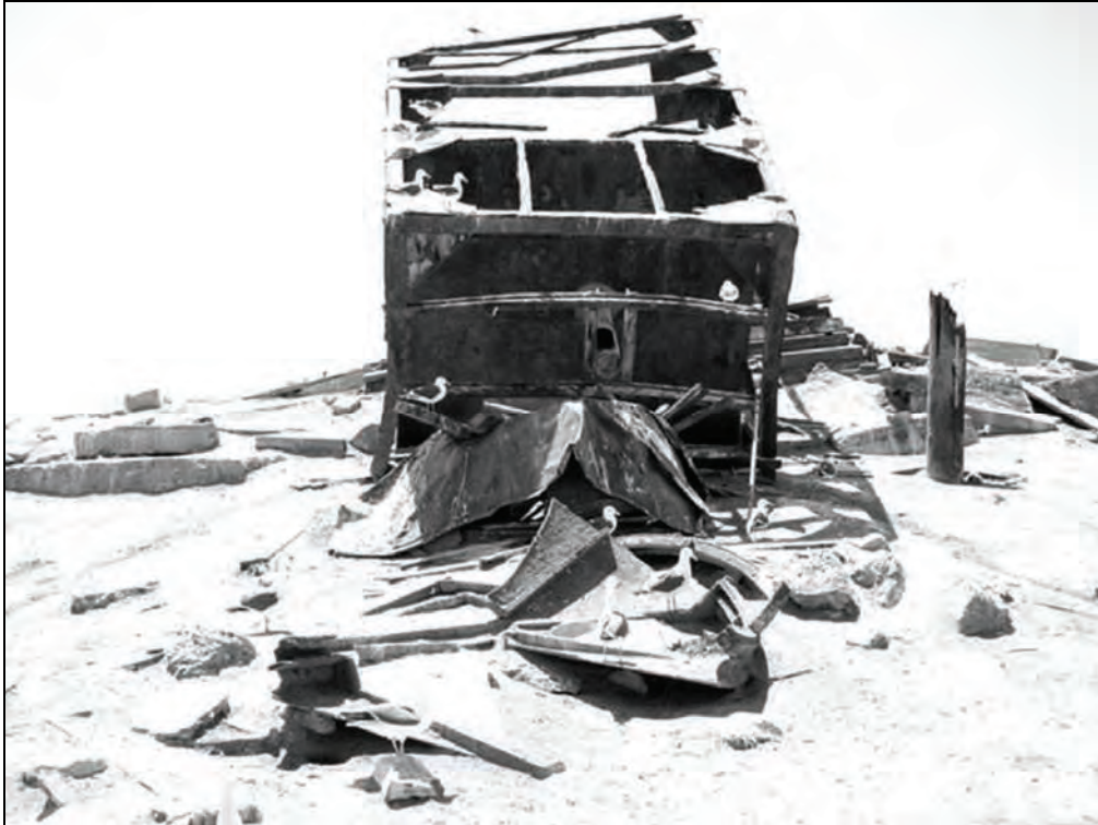
Figure 104. Steel Light Tower, 2005.
