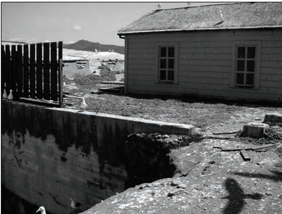
Figure 90. Retaining Wall Adjacent to 1881 Section of Fog Signal Building, looking West, 2005.
