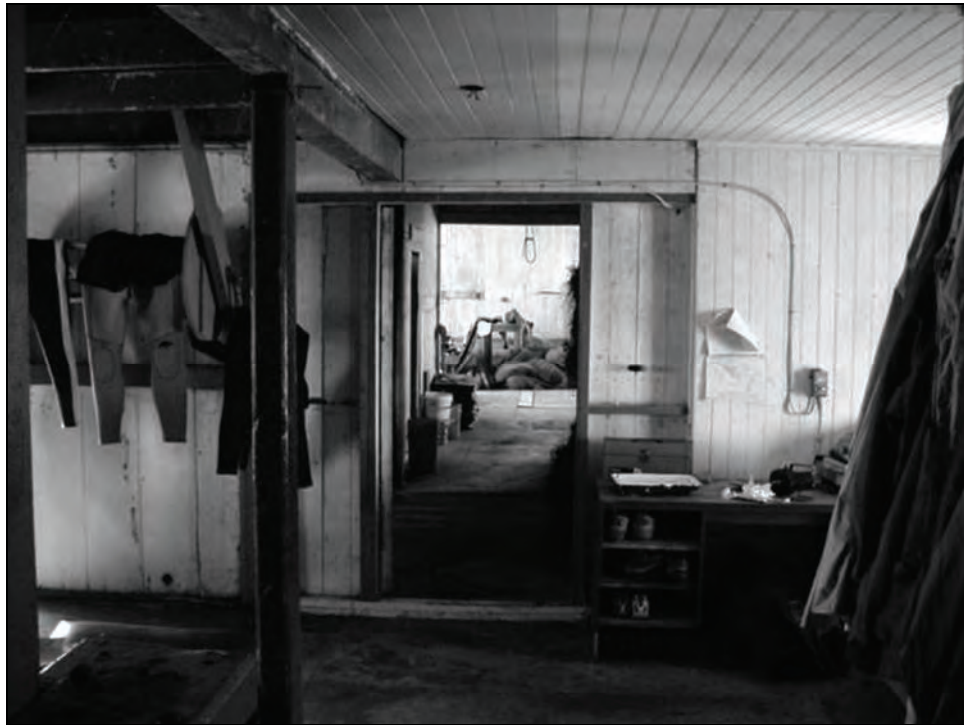
Figure 92. Interior of 1881 Section of Fog Signal Building, looking through Gallery (Southwest) to 1899 Building, 2005.
