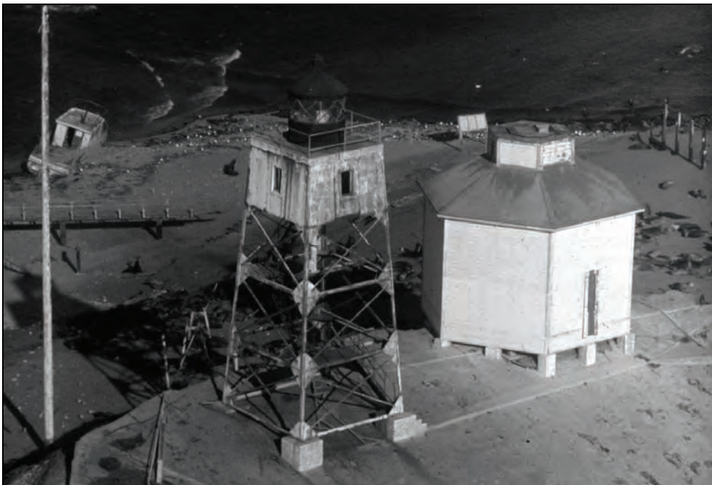
Figure 101. Steel Light Tower adjacent to Tank House, 1961.
