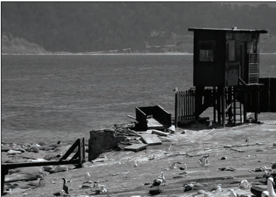
Figure 115. Foundation of Boathouse to left of Modern Blind, 2005.
