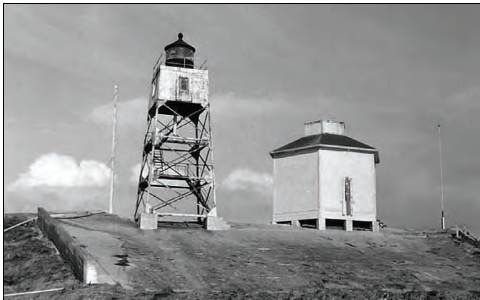
Figure 48. Steel Light Tower adjacent to Tank House, circa late 1940s.
