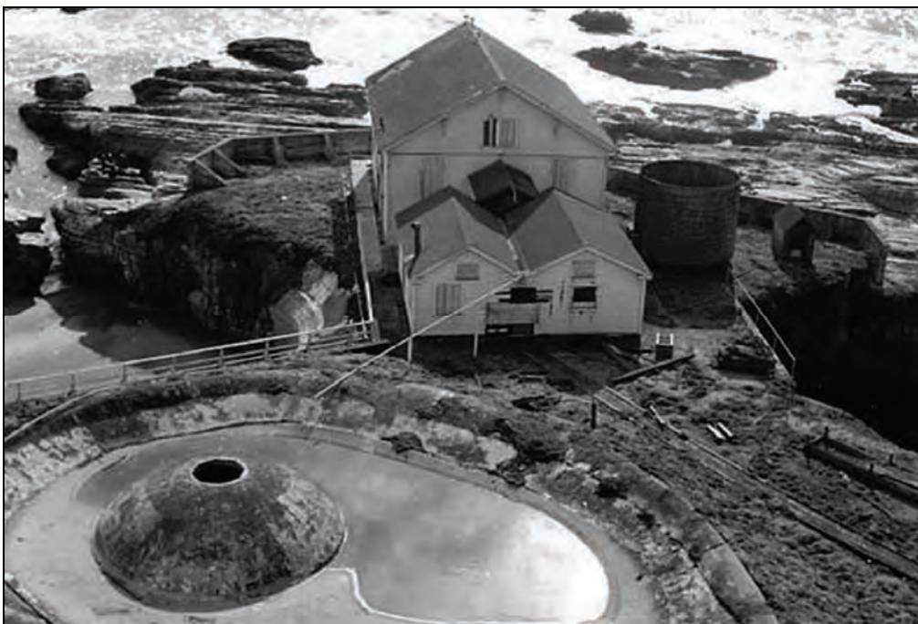
Figure 105. Fog Signal Building with Water Tank at Right, 1957.
