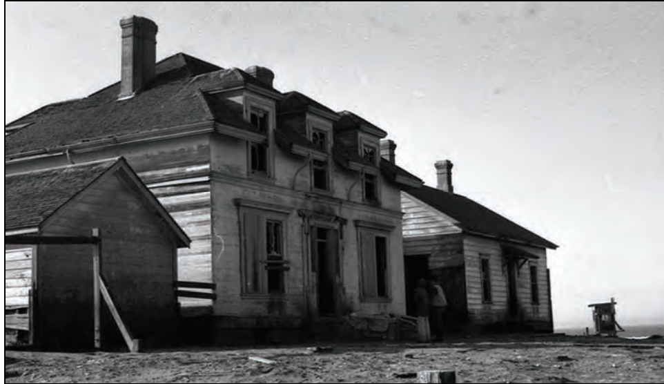
Figure 69. Front (east) of Keeper's Dwelling (Addition) in between Original at Right and Shed at Left, 1982.
