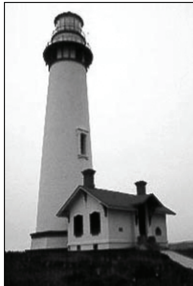
Figure 31. Pigeon Point Lighthouse showing attached Oil Room and Shop Structure.
