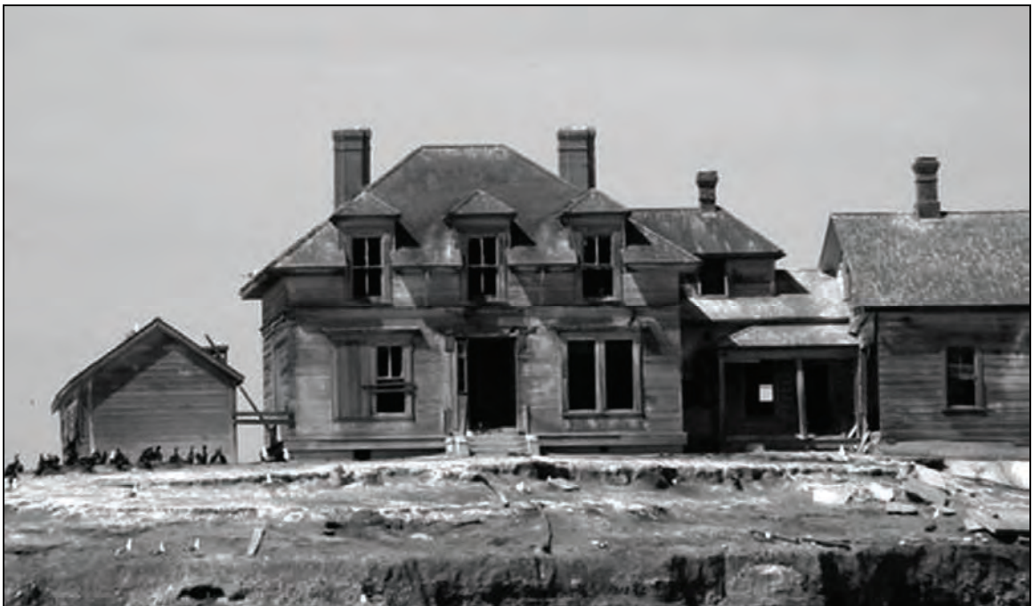
Figure 74. Keeper's Dwelling (1906 Addition), 2005.
