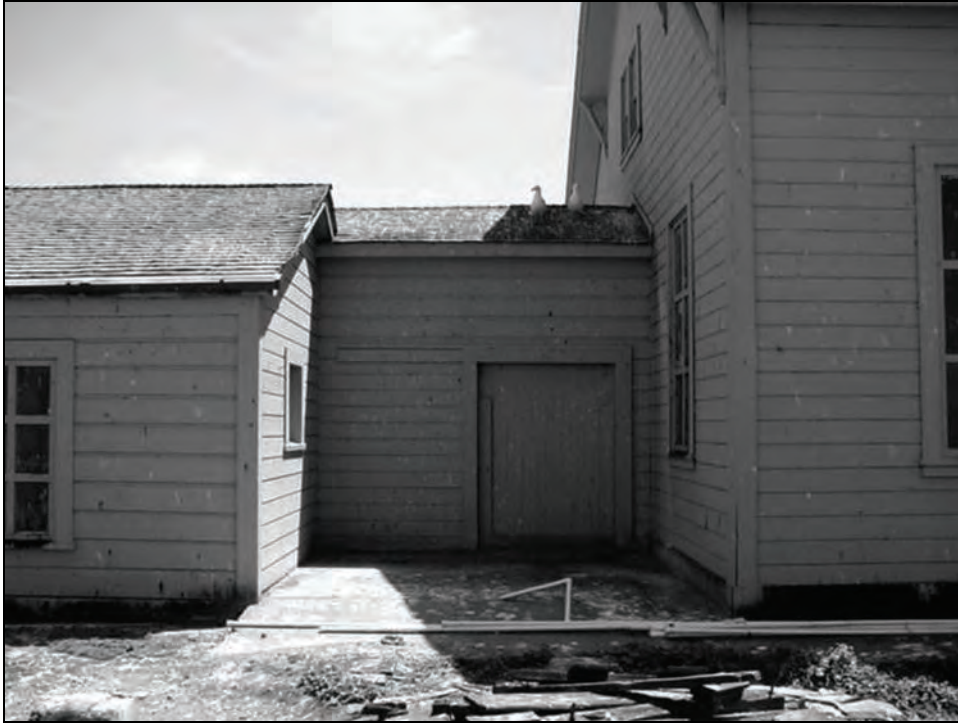
Figure 89. Fog Signal Building Gallery, 2005.
