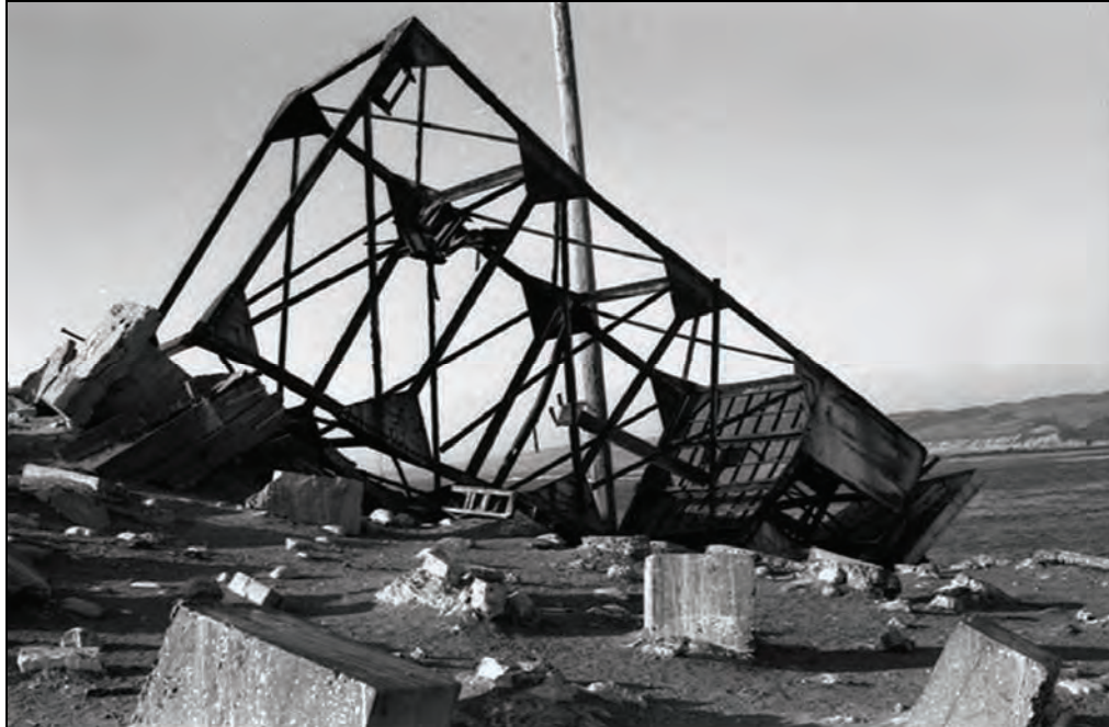
Figure 102. Steel Light Tower following Dismantling by State, 1982.
