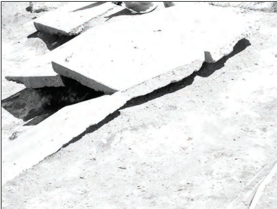
Figure 125. Remains of Concrete Walkway near Keeper's Dwelling, 2005.
