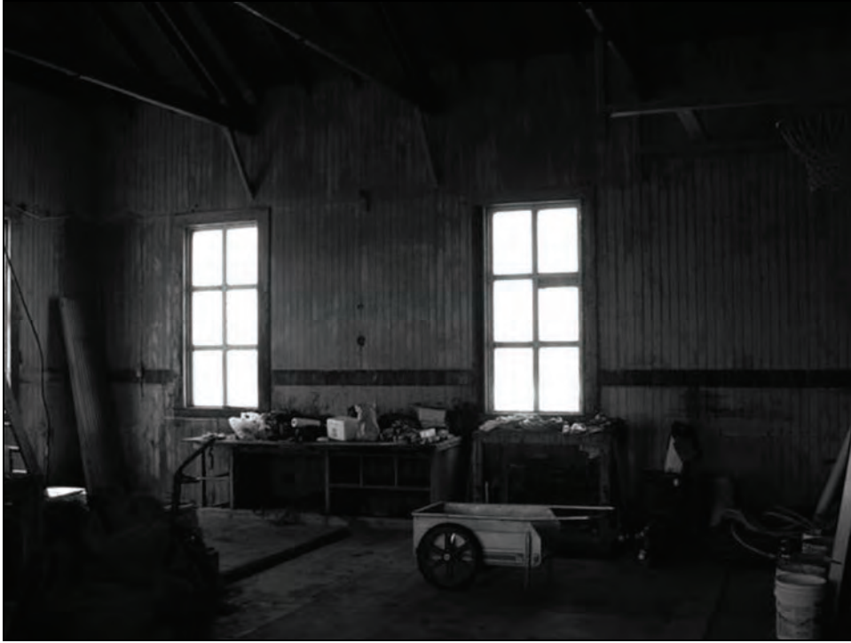
Figure 97. Interior of 1899 Fog Signal Building, Northwest Wall, 2005.
