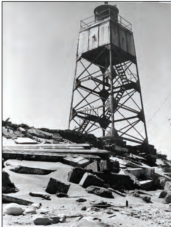
Figure 99. Steel Light Tower, ca. late 1950s.
