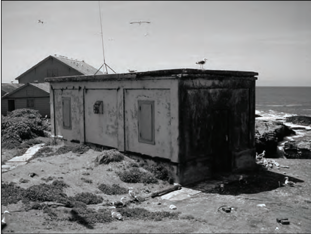
Figure 117. Fuel Storage/Paint Locker Building, looking Southwest, 2005.
