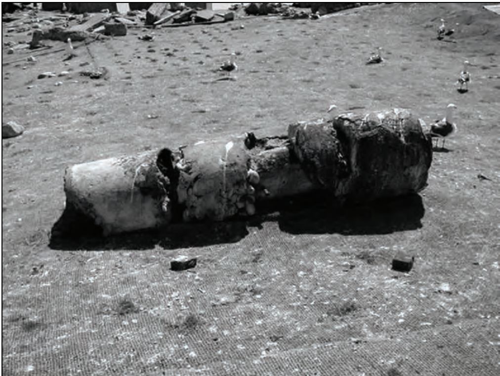
Figure 129. Concrete-encased Phone Pole, 2005.
