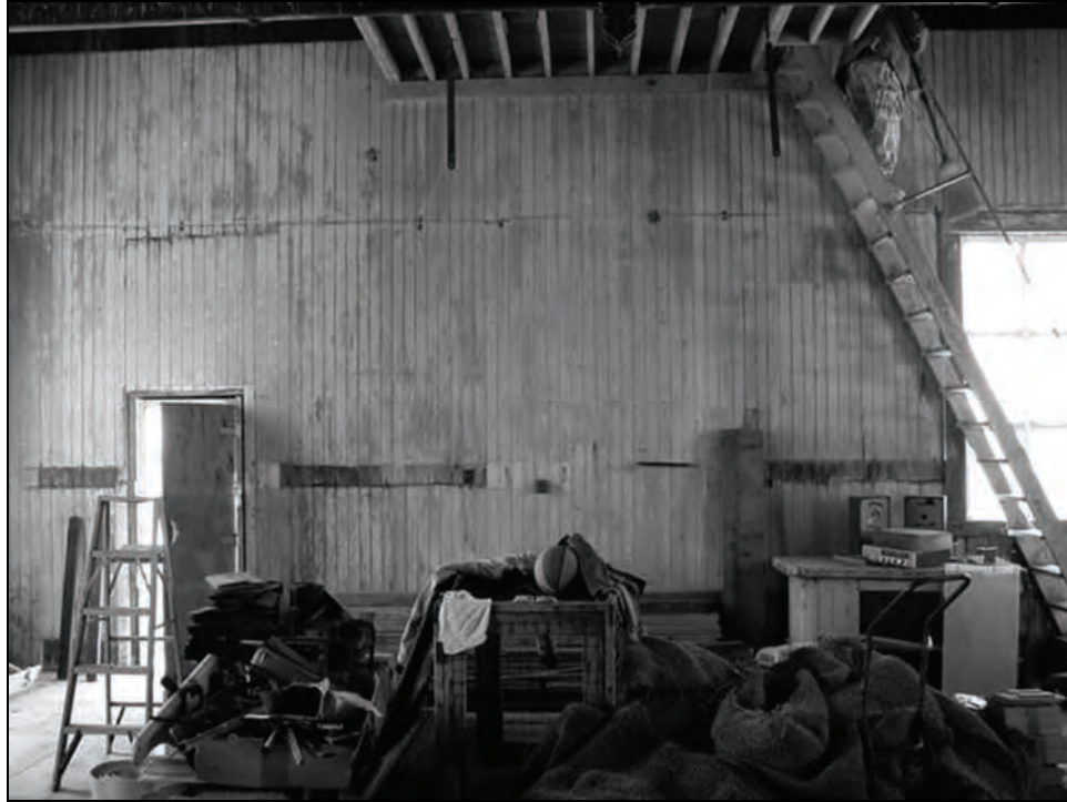
Figure 95. Interior of 1899 Fog Signal Building, Southwest Wall, 2005. Loft visible at top of photograph was original location of fog signal whistles.
