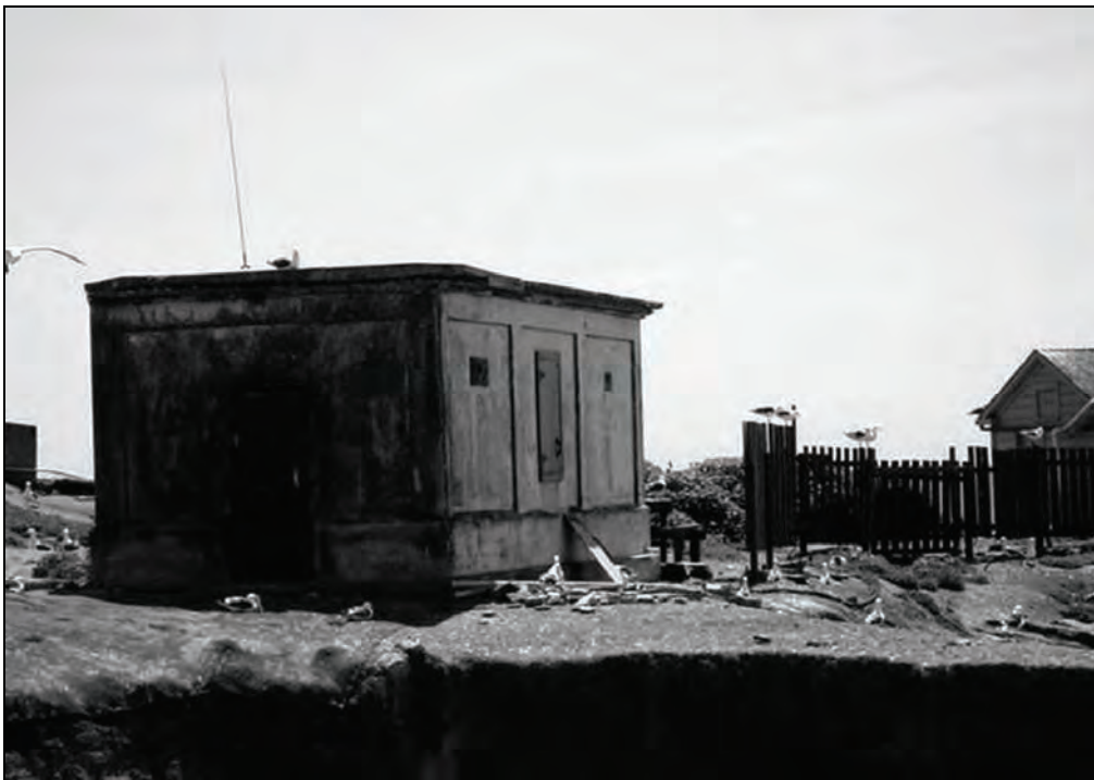
Figure 118. Fuel Storage/Paint Locker Building, looking Southeast, 2005.
