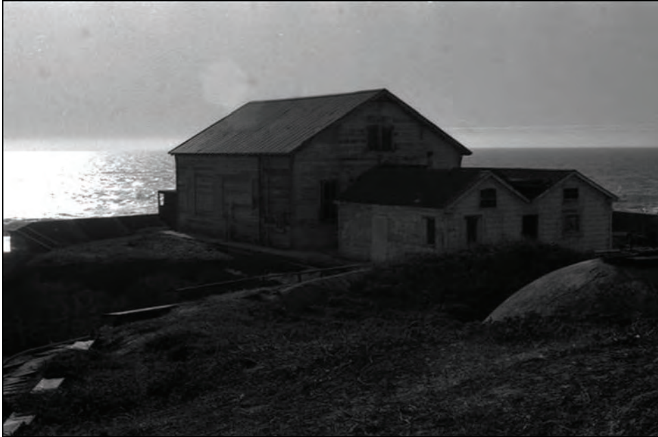
Figure 84. Fog Signal Building, 1982.
