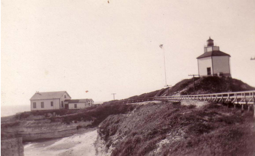
Figure 23. Wood walkway (catwalk) from keeper's dwelling to fog signal building (at left), light on tank house, 1926. Jack Chambers photograph, California State Parks
