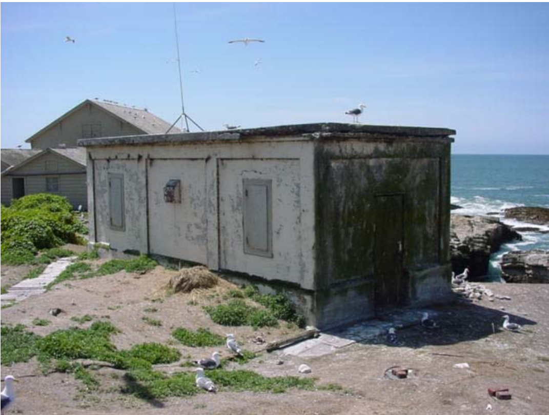
Figure 97. Fuel Storage/paint locker building, looking southwest, 2005.
