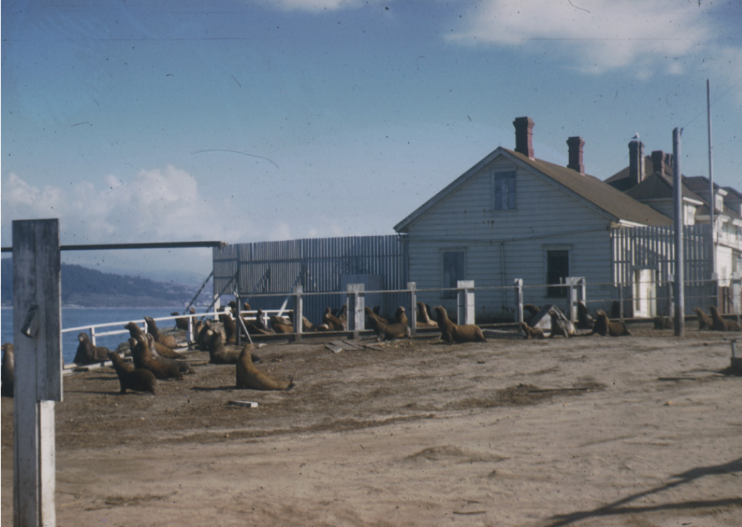
Figure 41. North end of assistant keeper's dwelling, ca. 1958. California State Parks
