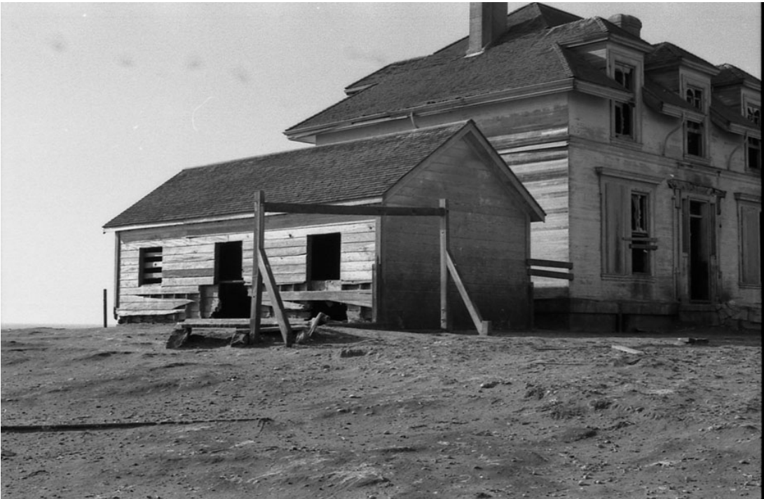
Figure 51. South end of keeper's dwelling with shed, 1982. Catalog #24743, California State Parks, Archaeology Laboratory, West Sacramento.
