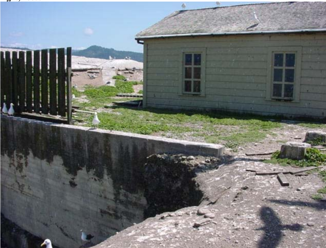
Figure 69. Retaining wall adjacent to 1881 section of fog signal building, looking west, 2005.
