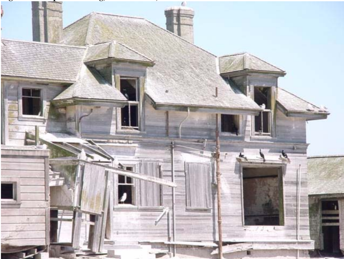
Figure 53. Keeper's dwelling (1906 addition), 2005.
