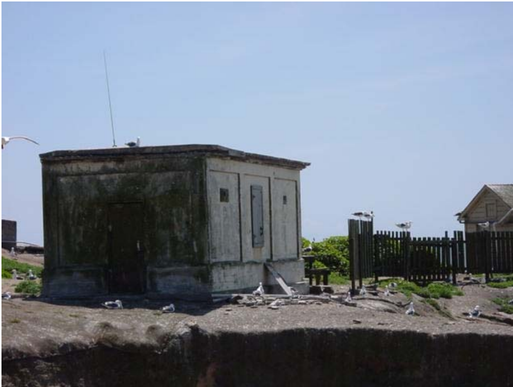
Figure 98. Fuel Storage/paint locker building, looking southeast, 2005.
