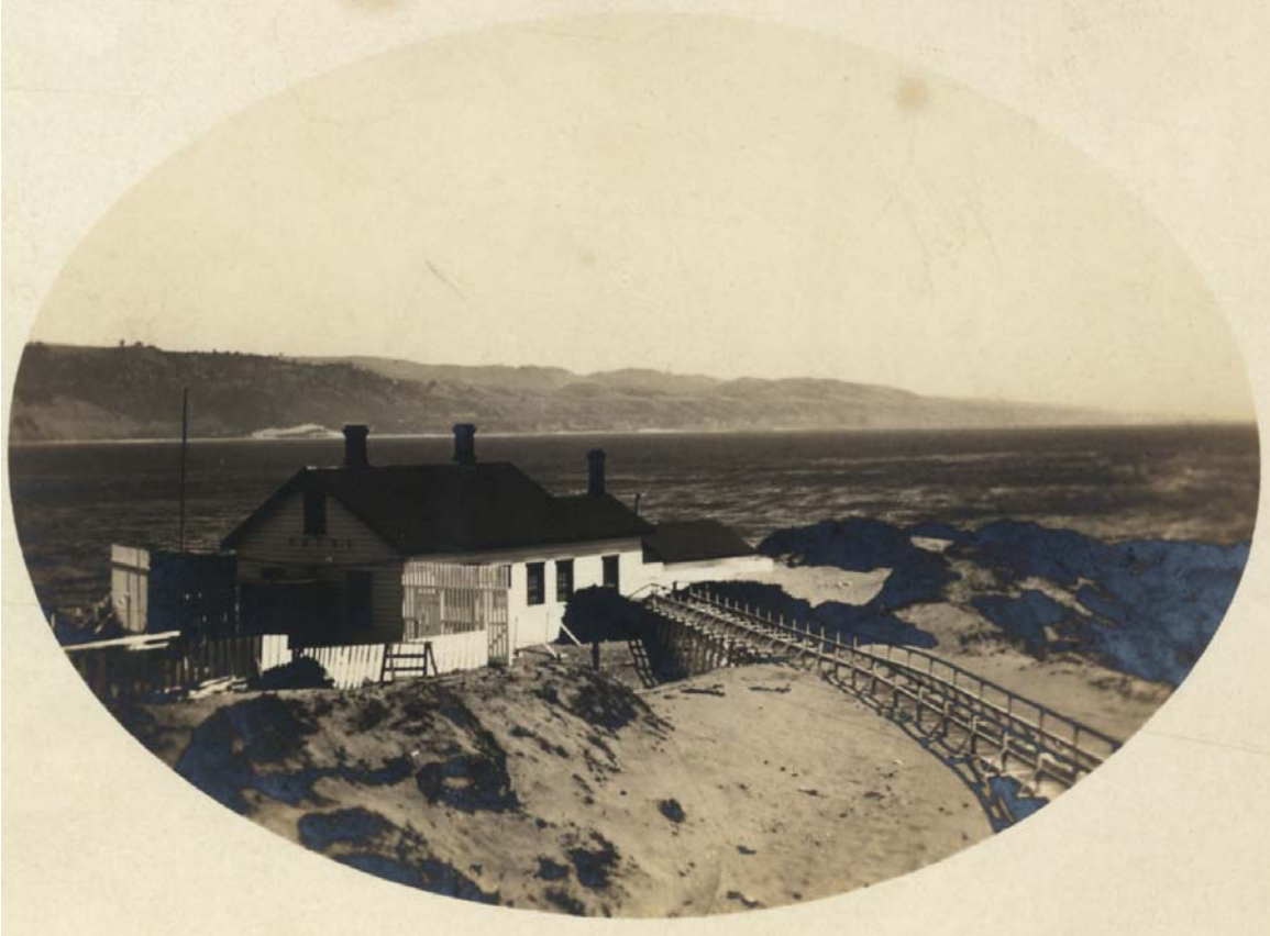
Figure 63. Fog signal building looking south, unknown date. Note tramway at right and fences adjacent to building. Courtesy of Department of Special Collections, Stanford University Libraries.
