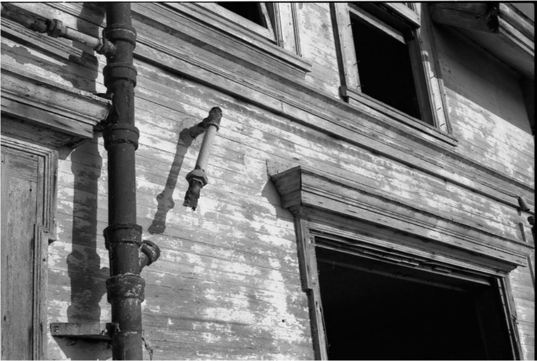
Figure 49. Exterior of west wall, keeper's dwelling (1906 addition), showing broken iron pipes, window frames, and molding, 1982. Catalog #24736, California State Parks, Archaeology Laboratory, West Sacramento.
