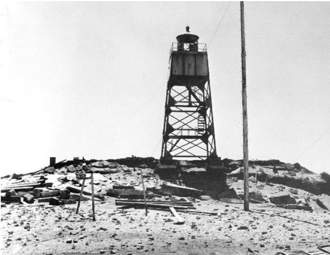
Figure 34. Steel light tower shortly before being cut down. California State Parks
