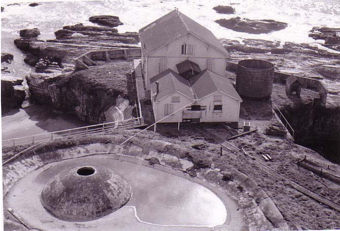
Figure 57. Fog signal building with water tank and distillate house to the right. Second (1881) fog signal building is twin gable structure at rear of larger building (1899). Water shed and cistern are in foreground. Seawall is visible at front, 1957. California State Parks
