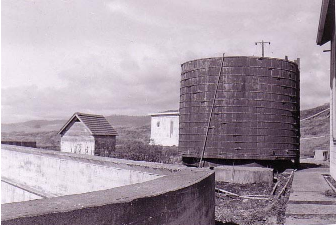
Figure 86. Water tank adjacent to fog signal building, 1957. Concrete retaining wall is visible in left foreground, Oil storage house and paint locker in rear, California State Parks.
