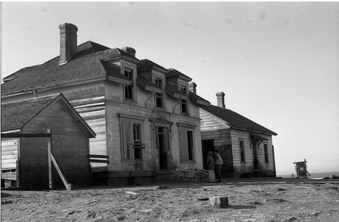
Figure 47. Front (east) of keeper's dwelling (addition) in between original dwelling at right and shed at left, 1982. Catalog #24738, California State Parks, Archaeology Laboratory, West Sacramento.
