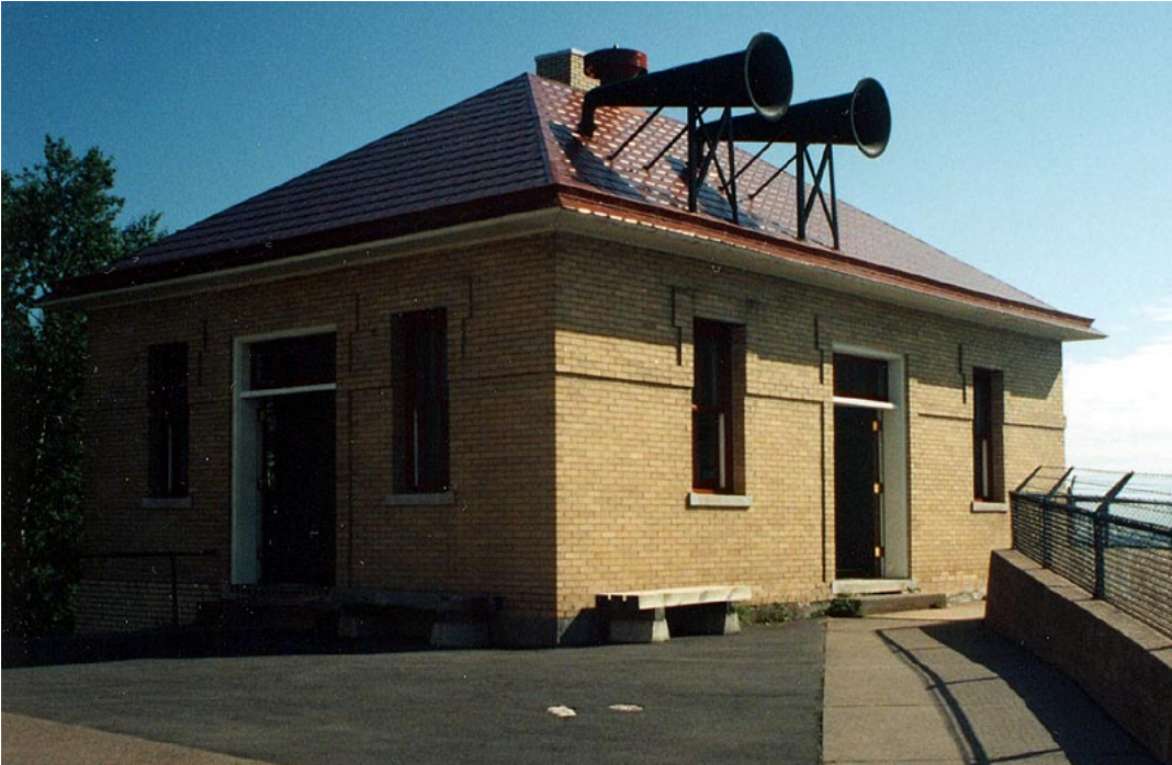
Figure 10. Fog horn building at Split Rock Light Station, Minnesota. Photograph by Dave Wobser.
