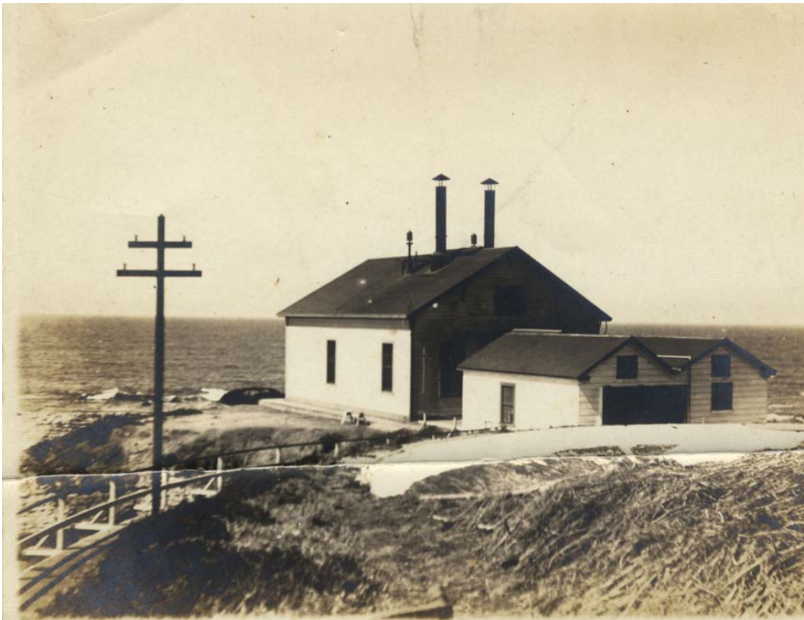
Figure 64. Fog signal building looking north, unknown date. Note sliding door on front of 1881 building. Fog signal whistles are visible on 1899 building. Courtesy of Department of Special Collections, Stanford University Libraries.
