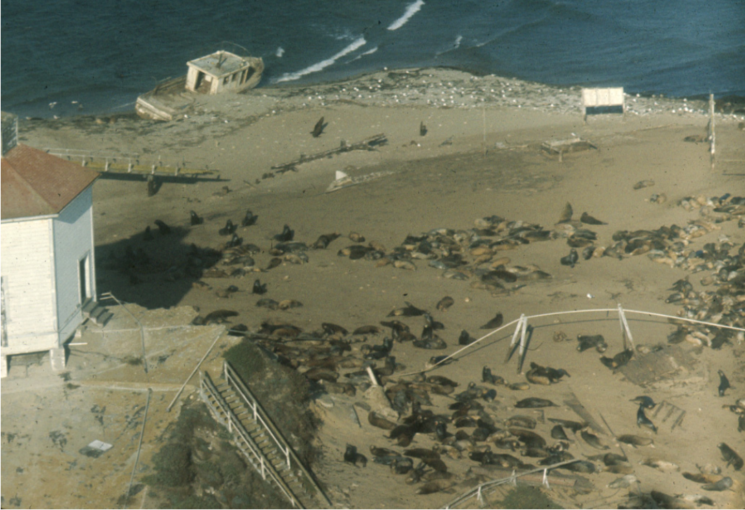
Figure 104. Portion of water tank structure, with wood stairway leading up to it, ca. 1961. California State Parks.
