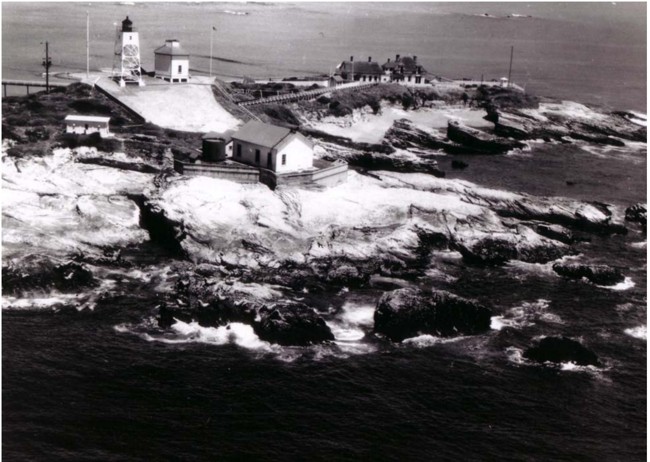
Figure 78. Overview of light station with light tower visible at left, 1953. U.S. Coast Guard photograph, U.S. Coast Guard Historian's Office, Washington, D.C. Note fog whistles are missing from gable end of fog signal building (replaced by automated system)
