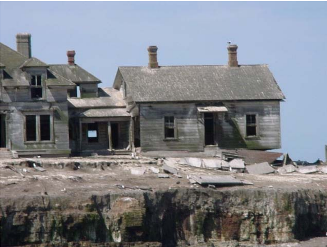
Figure 42. Keeper's dwelling, original portion on right, 1906 addition on left, 2005.
