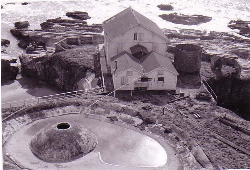
Figure 22. Fog Signal building with water tank and distillate house to the right. Water shed and cistern are in foreground. Seawall is visible at rear of fog signal building, 1957. California State Parks
