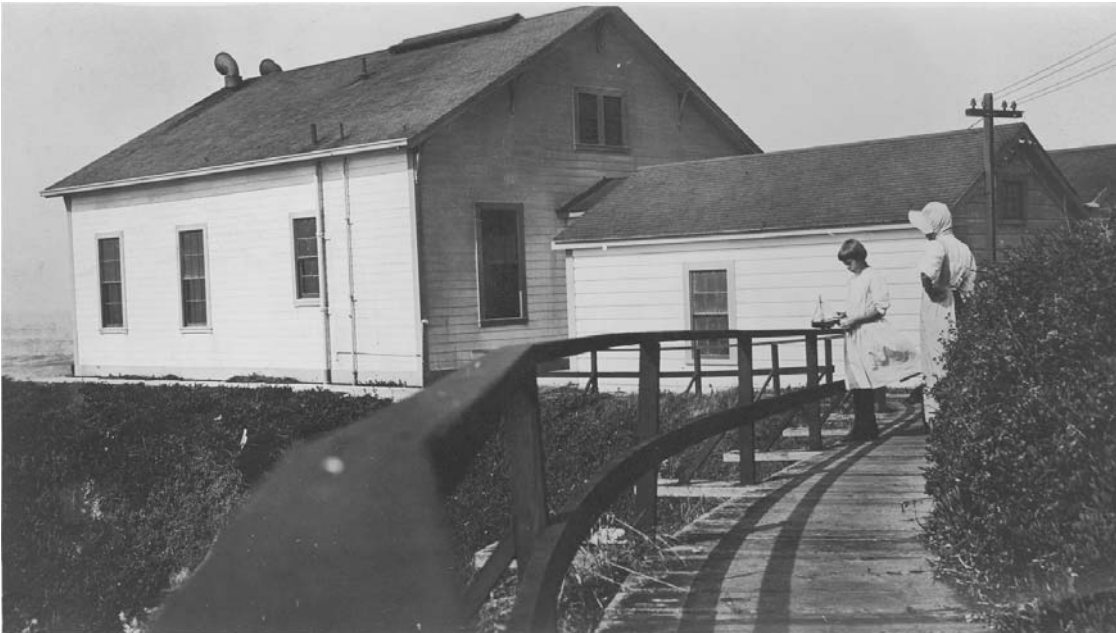
Figure 60. Fog signal building and wood walkway, ca. early 1920s. Note fog signals in gable end at left. Courtesy, U.S. Lighthouse Society, San Francisco, California.
