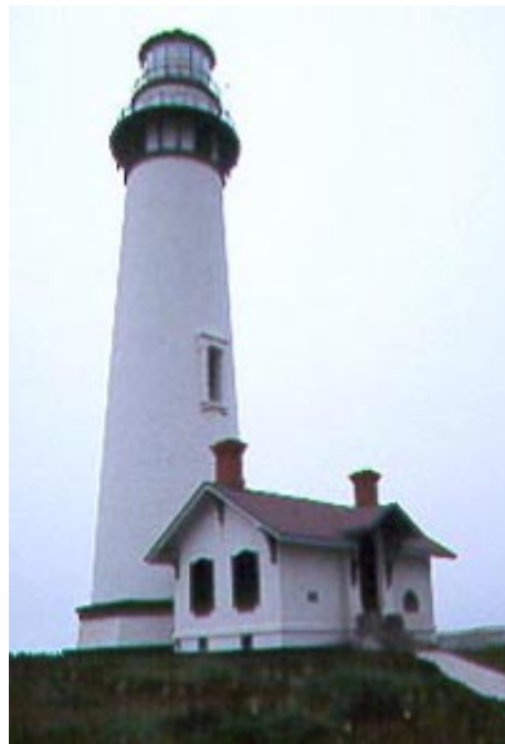
Figure 8. Pigeon Point Lighthouse showing attached oil room and shop structure. California State Parks
