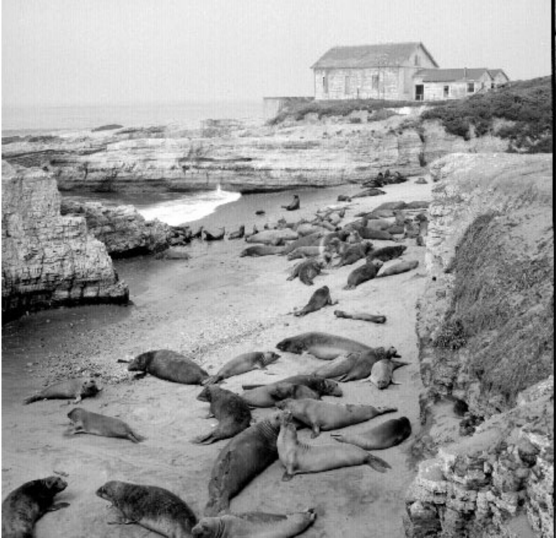
Figure 61. Fog signal building in background with seawall visible to left, 1966. California State Parks
