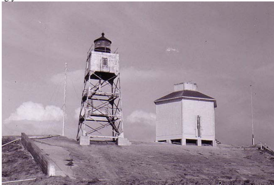
Figure 24. Steel light tower adjacent to tank house, ca. late 1940s, California State Parks
