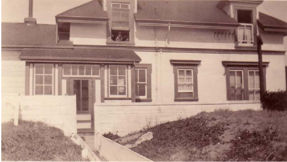
Figure 46. Rear (west) of keeper's dwelling (1906 addition), 1926. Jack Chambers photograph, California State Parks.
