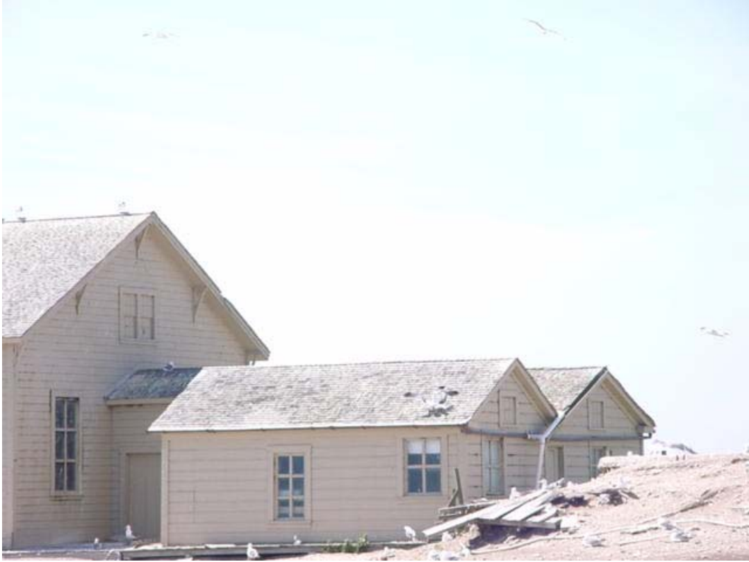
Figure 66. Fog signal building looking northwest, 2005.
