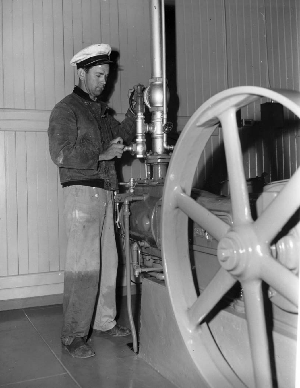
Figure 28. U.S. Coast Guardsman working on air compressor in Fog Signal Building, 1948. Reginald McGovern photograph, courtesy, U.S. Lighthouse Society, San Francisco, California.
