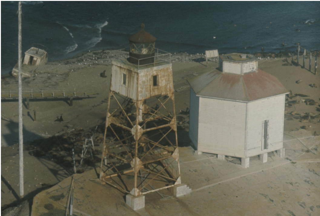
Figure 81. Steel light tower adjacent to tank house, 1961, California State Parks
