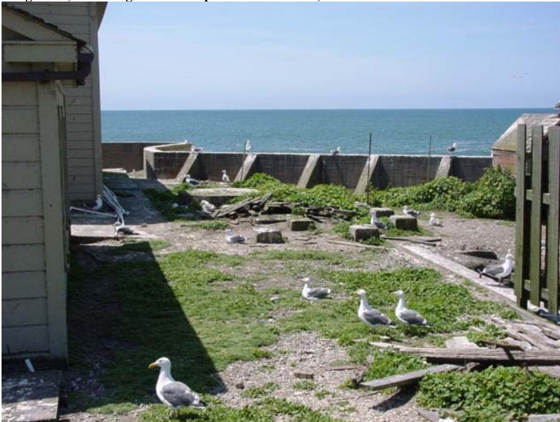
Figure 87. Foundation for water tank adjacent to fog signal building, 2005. Concrete retaining wall is visible at rear.
