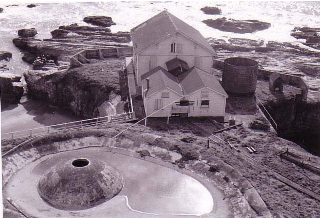
Figure 85. Fog signal building with water tank at right, 1957. California State Parks
