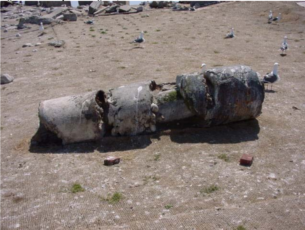
Figure 108. Concrete encased phone pole, 2005.
