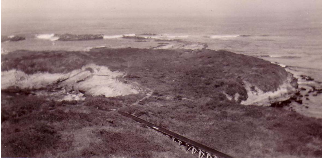
Figure 18. Portion of tramway at north end of island in 1926. Jack Chambers photograph, California State Parks
