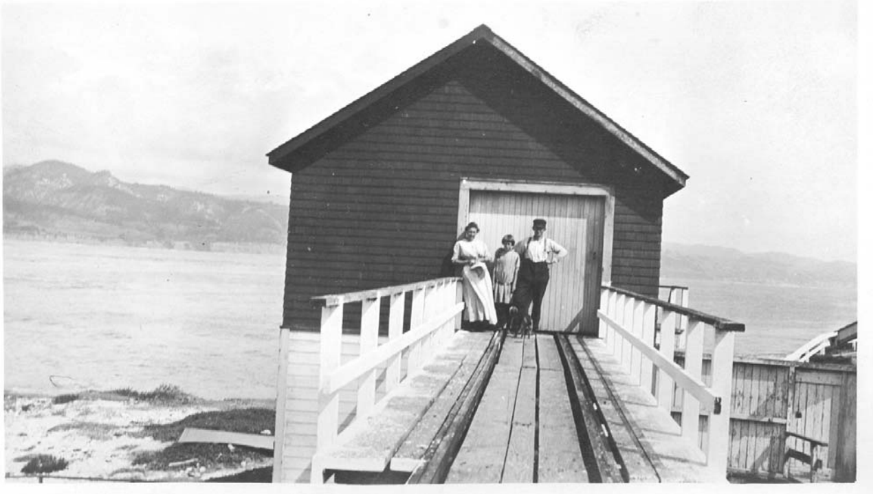
Figure 93. Boathouse at end of tramway, unknown date. Courtesy, U.S. Lighthouse Society, San Francisco, California.
