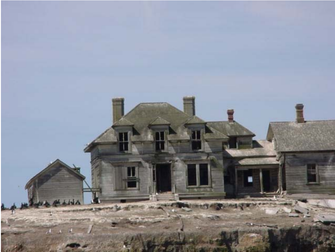
Figure 52. Keeper's dwelling, 1906 addition, 2005.
