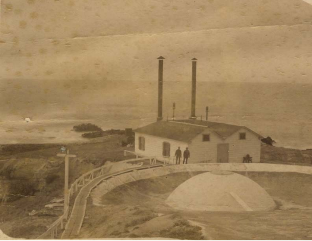
Figure 56. Second fog signal building (built 1881) in front of water-shed and cistern, ca. late 1880s. Fog whistles are smaller vertical members protruding from roof. Larger pipes are vents for boilers. Note similarity to fog signal building at Pigeon Point in Figure 11. Courtesy of Department of Special Collections, Stanford Libraries.
