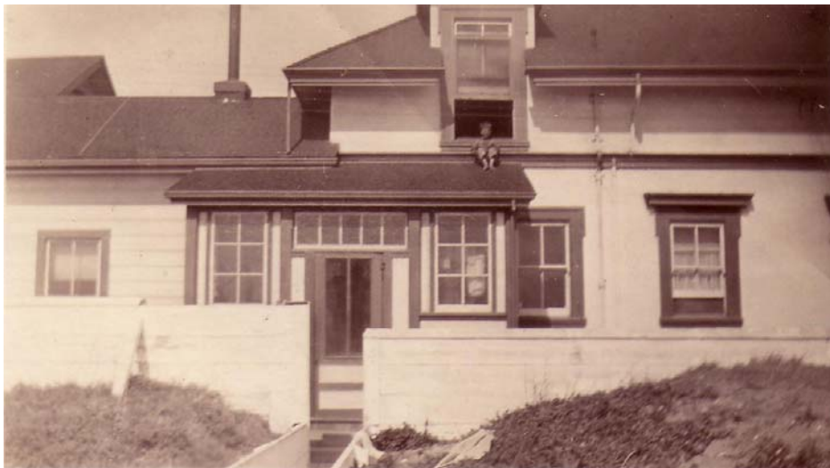
Figure 45. Rear (west) of keeper's dwelling (1906 addition), showing separation between original building (on left), and addition on right, 1926. Jack Chambers photograph, California State Parks.
