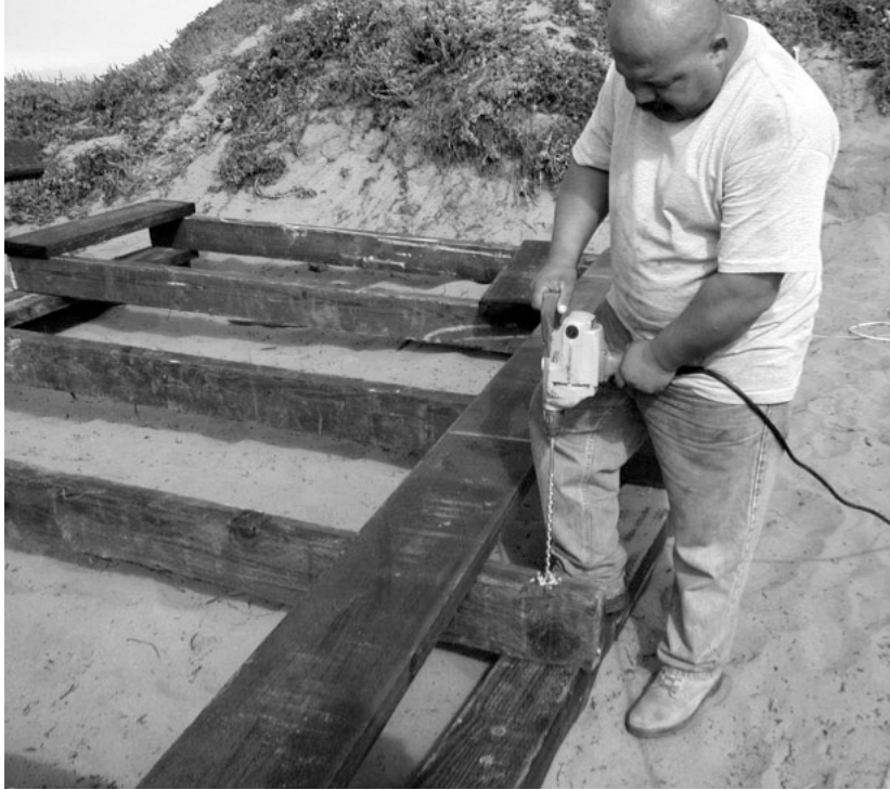
Figure 33. Drilling Stringers for Metal Rebar Anchor Pins.
