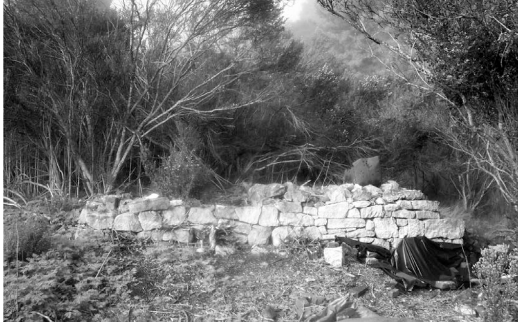
Figure 68. Feature C, East Wall.
