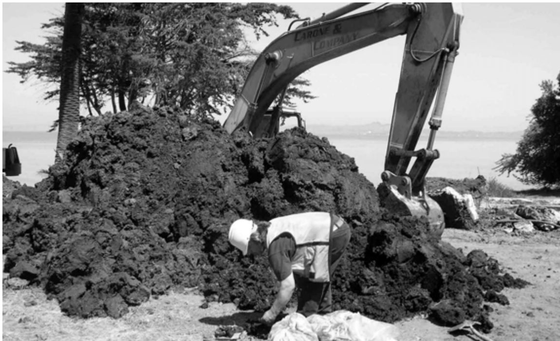
Figure 19. Stockpiled Soils from Buried Component, Locus C, Trench 13.
