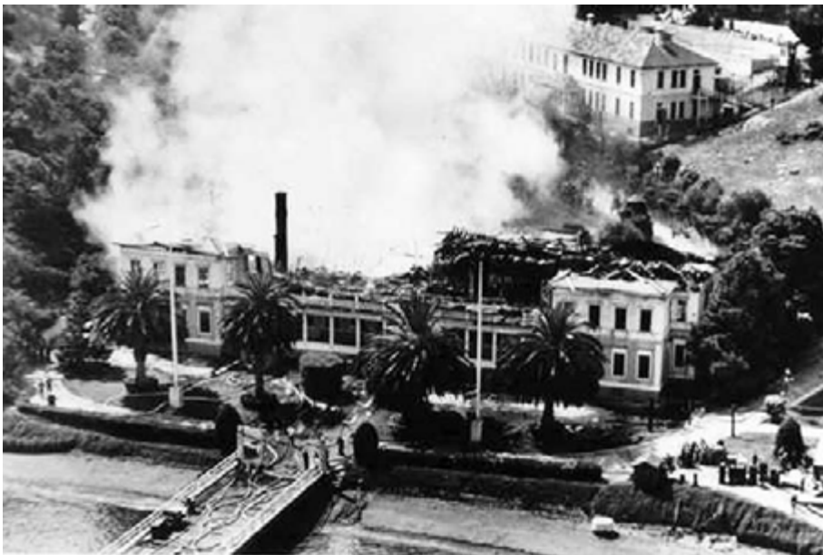
Figure 6. Fire in the Administration Building 1940 (CDPR Archives).
