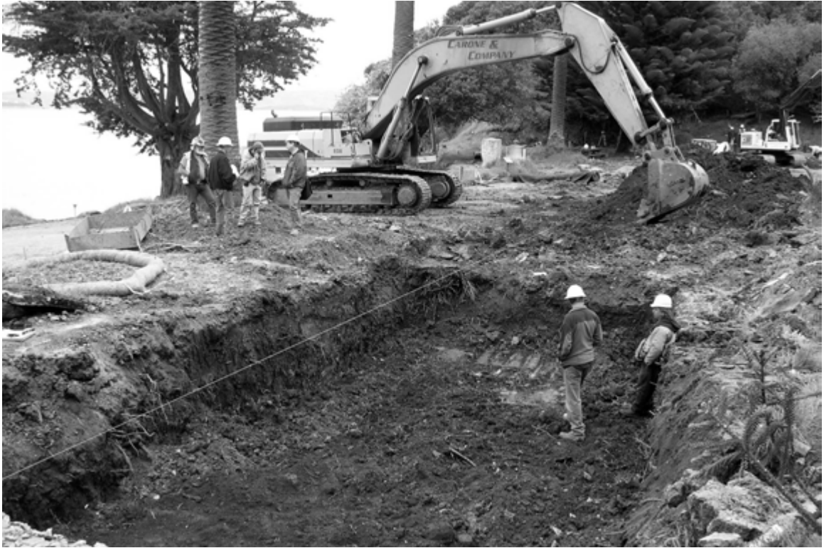
Figure 17. Septic Tank Exposure, Locus B.
