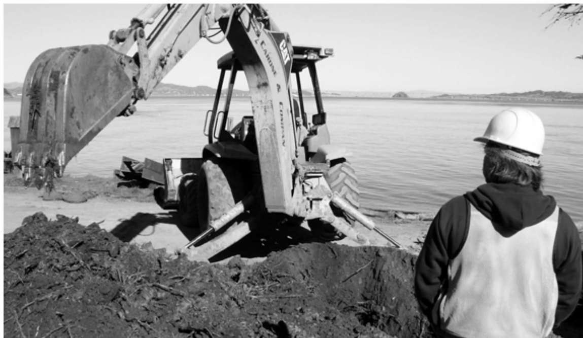
Figure 16. Mechanical Trenching Areas of Proposed Impacts.
