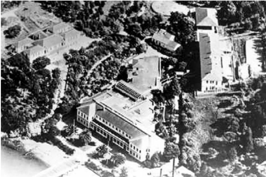
Figure 5. Aerial View of Immigration Station Complex circa 1910 (CDPR Archives).
