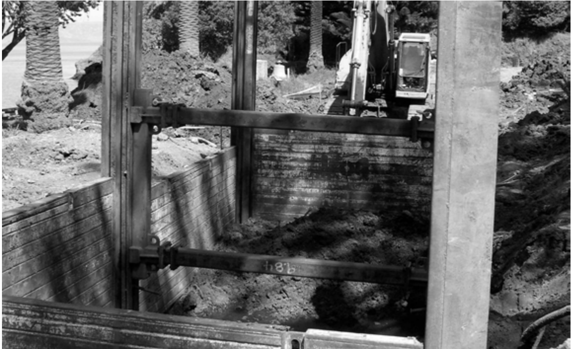
Figure 21. Septic Tank Exposure with Trench Plate Shoring, Locus B.
