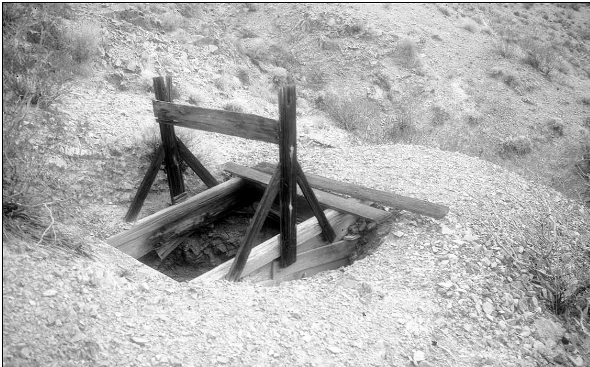
Figure 19. Shaft (SM-06) with Windlass at Santa Monica Gulch Mining Complex.
