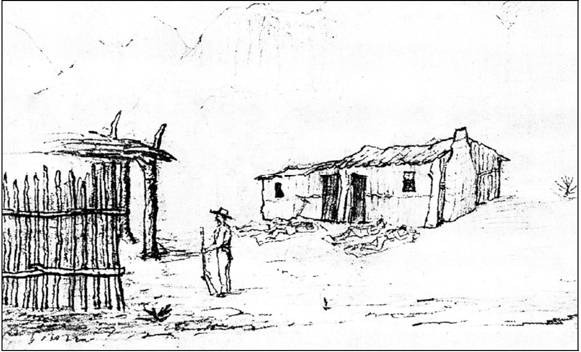
(a) Thatch Roof Wattle and Daub House with Wood Stockade Corral, Fort Davis, 1858 (original drawing by Phocion Way, reproduction courtesy of the Journal of the Southwest , University of Arizona).
