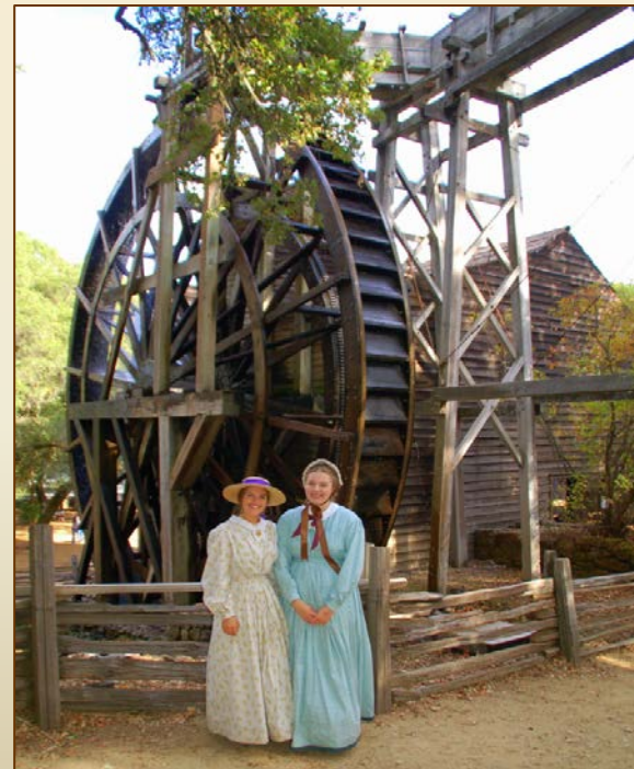
Bale Grist Mill SHP Napa County Regional Park and Open Space District
