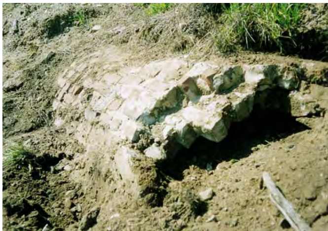
Remnants of the Zanja Madre or “Mother Trench” that first brought water from the Los Angeles River to El Pueblo de Los Angeles in 1781 have been found at the Cornfield. 10
