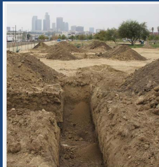
The Dig Begins
