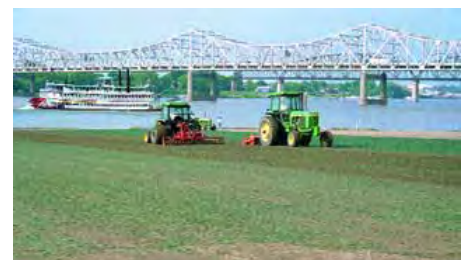
Tilling reinforcing fibers into the soil
