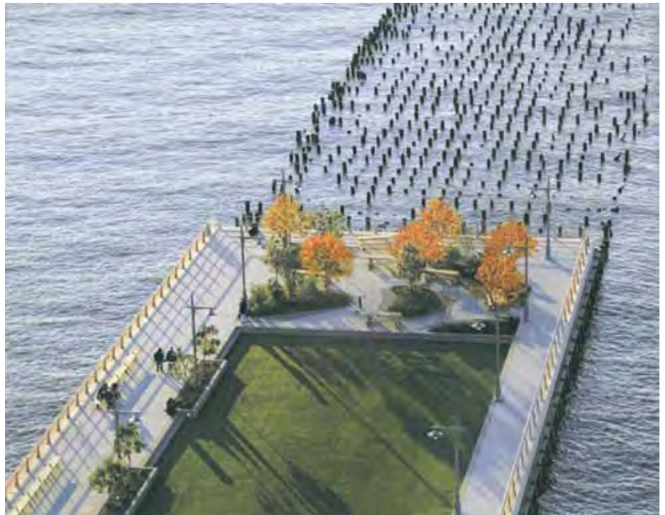
Precedent - Pier promenade and picnic area with remnant pilings
