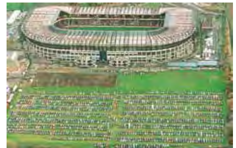
Precedent - Fiber-reinforced turf at Murray Field Stadium, Scotland
