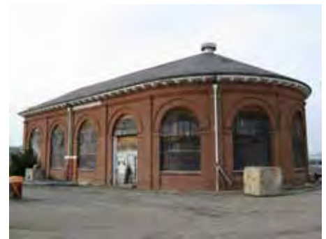
Pumphouse at Drydock 3
