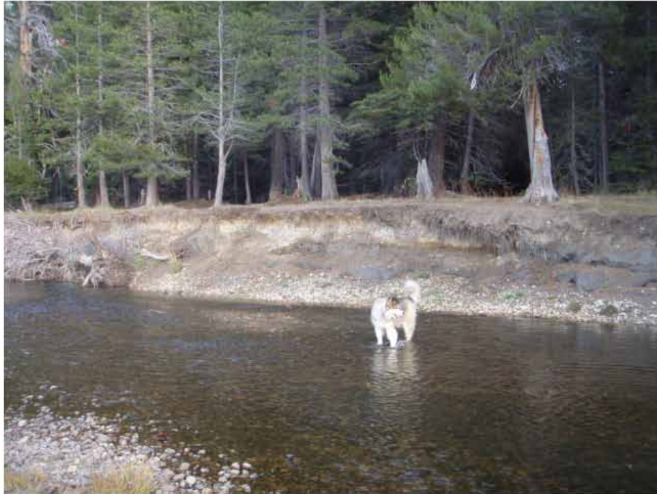
Eroding Bank at RS 9300
